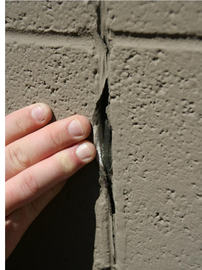
Adhesive Failure
