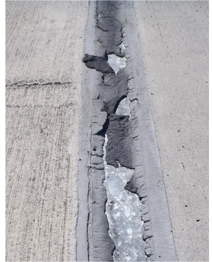
Expansion Joint Failure
