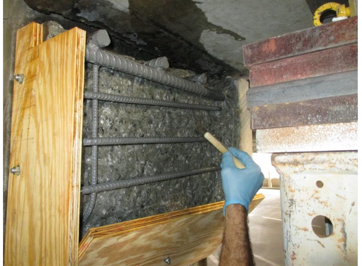
Applying Epoxy Bonding Agent
