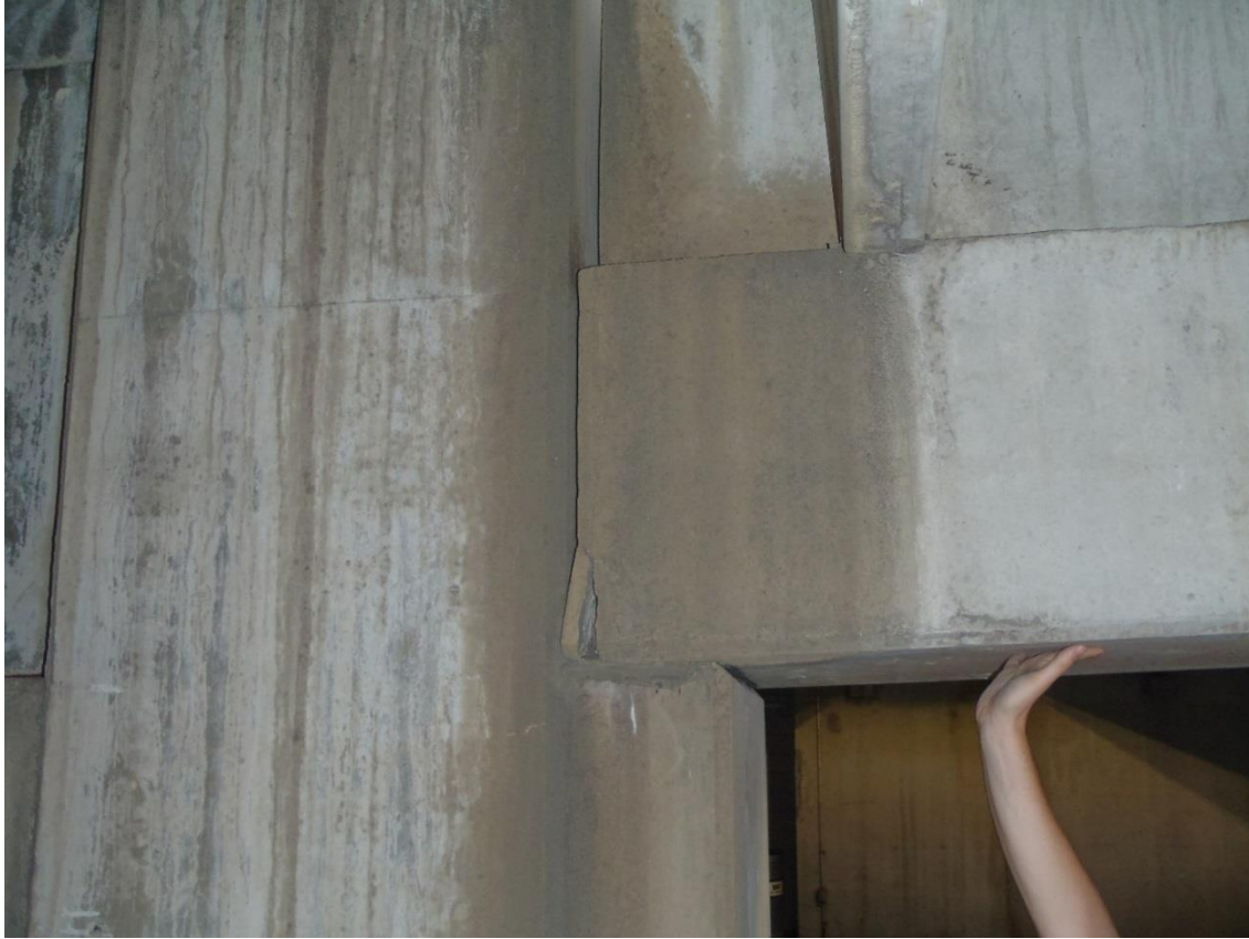
Precast Beam Haunch
