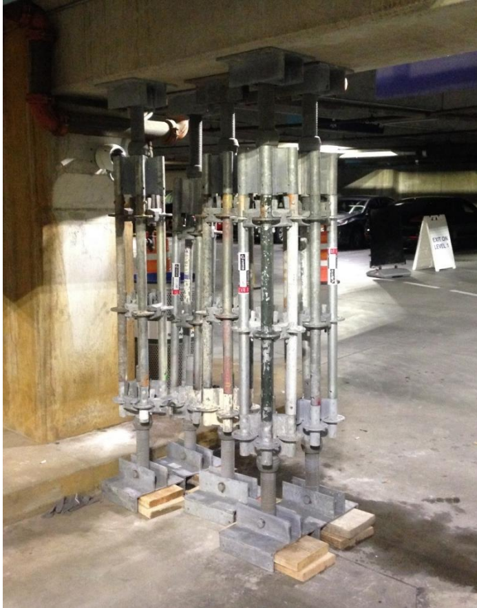
Shoring to Remove Load
