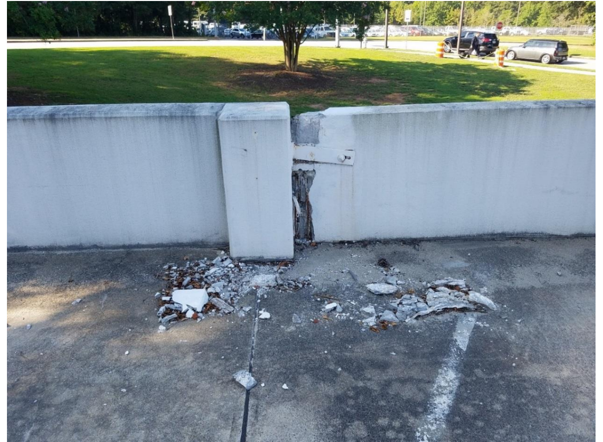
Broken Precast Spandrel Beam
