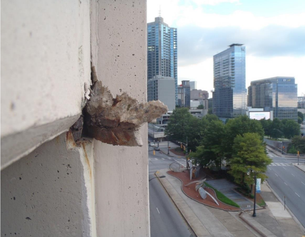
Spall Over Sidewalk
