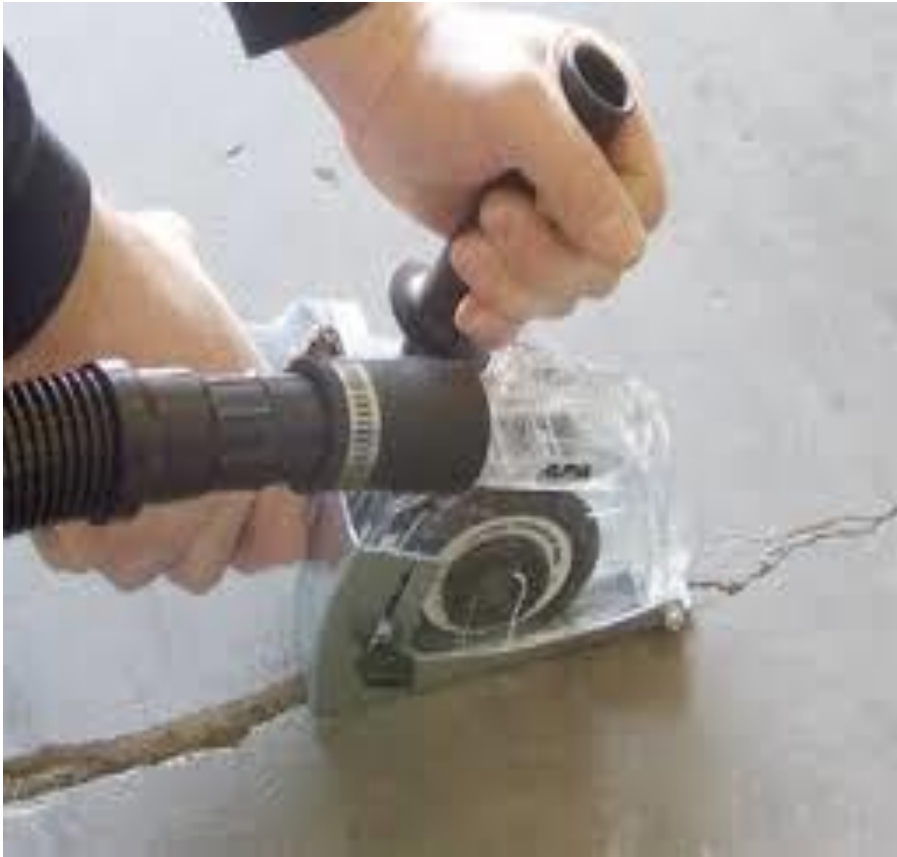
Crack Chasing
