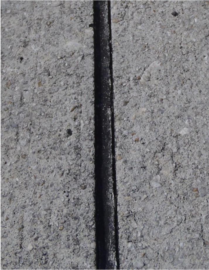
Sealant Failure
