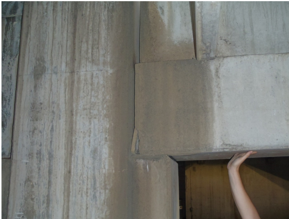
Precast Beam Haunch
