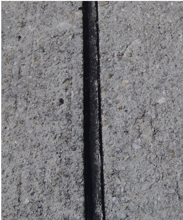
Sealant Failure
