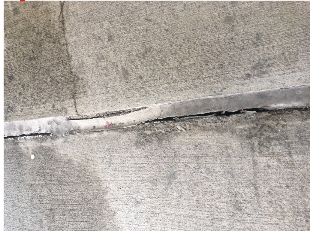
Adhesive Failure
