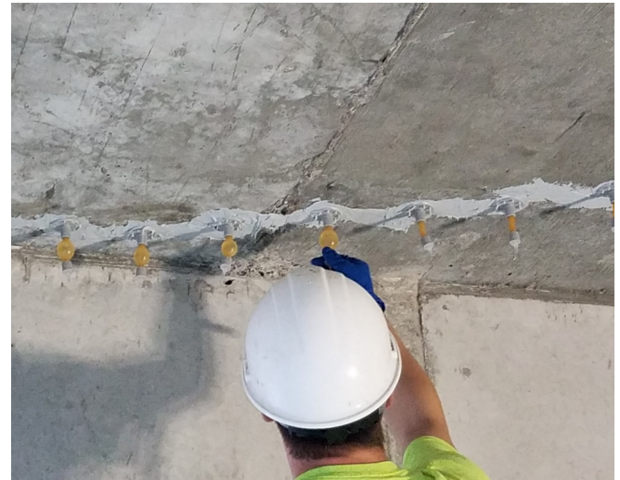
Inflatable Injection Port
