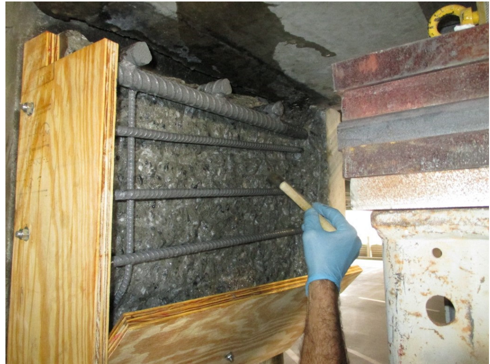
Applying Epoxy Bonding Agent
