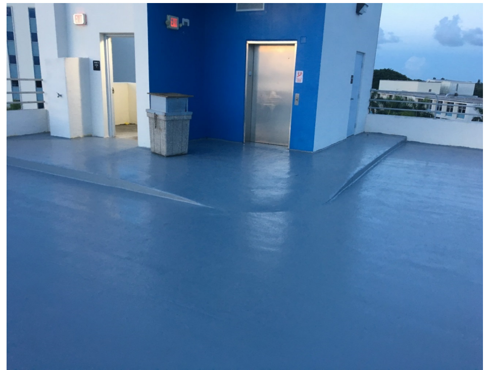
Traffic Bearing Membrane
