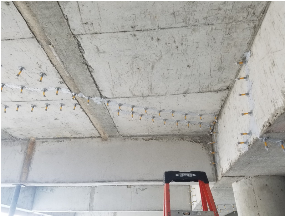
Cracks \geq .035"
