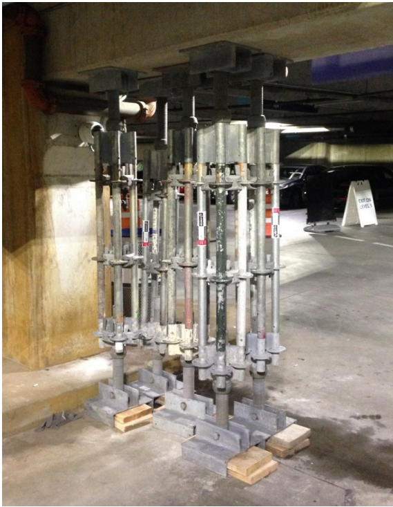
Shoring to Remove Load
