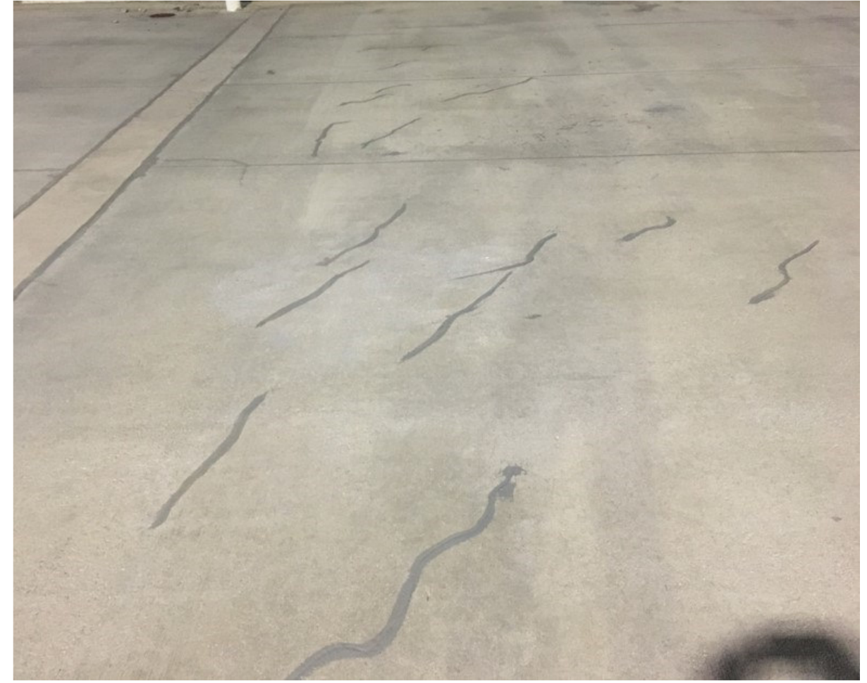
Crack Sealant
