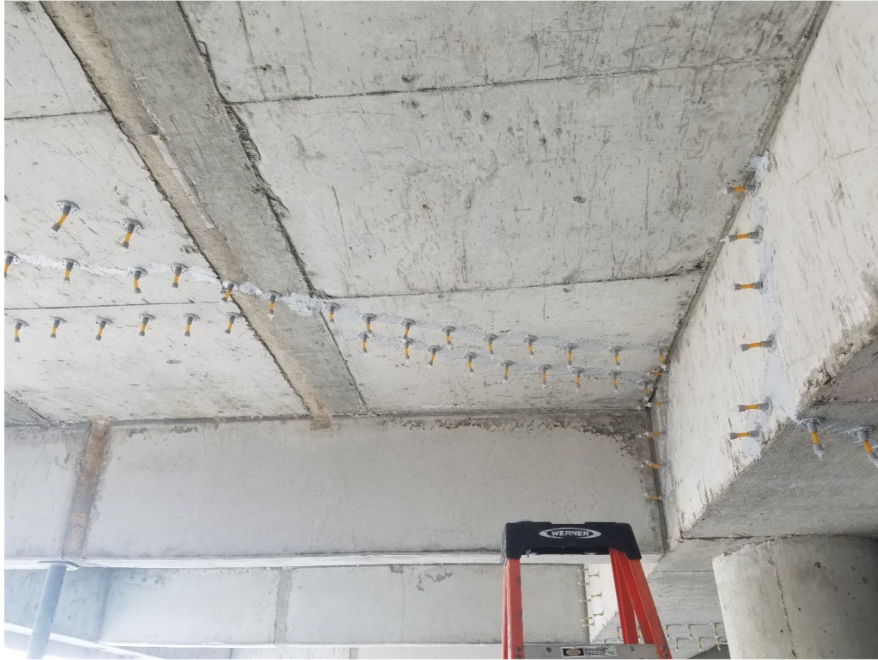
Cracks \geq .035"
