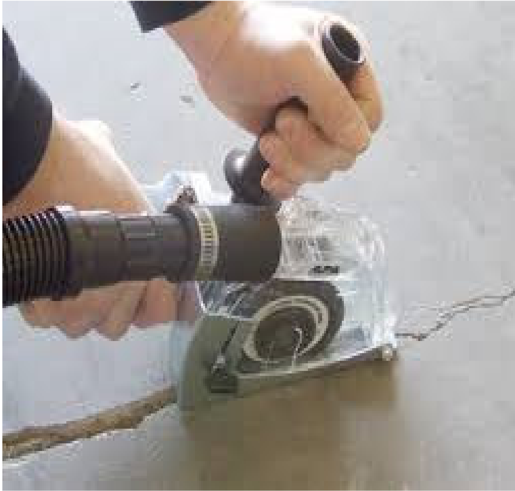
Crack Chasing
