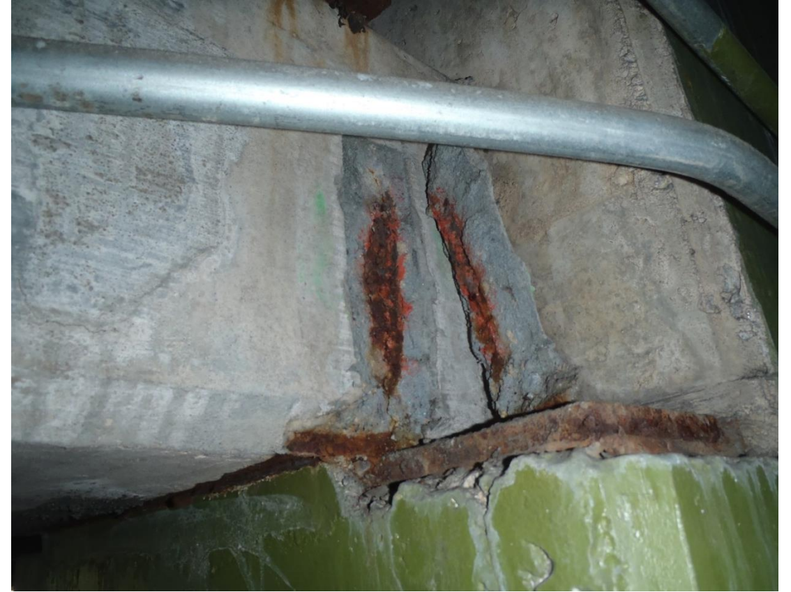
Improper Surface Preparation
