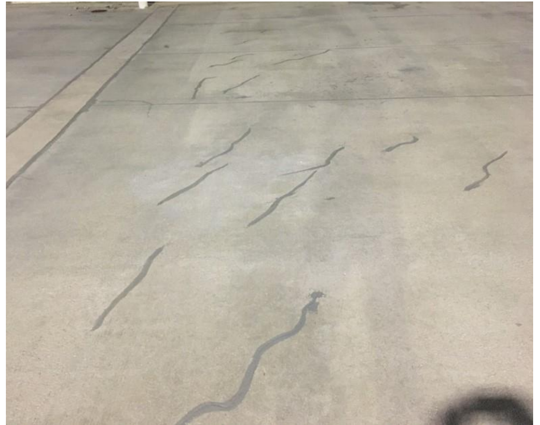
Crack Sealant
