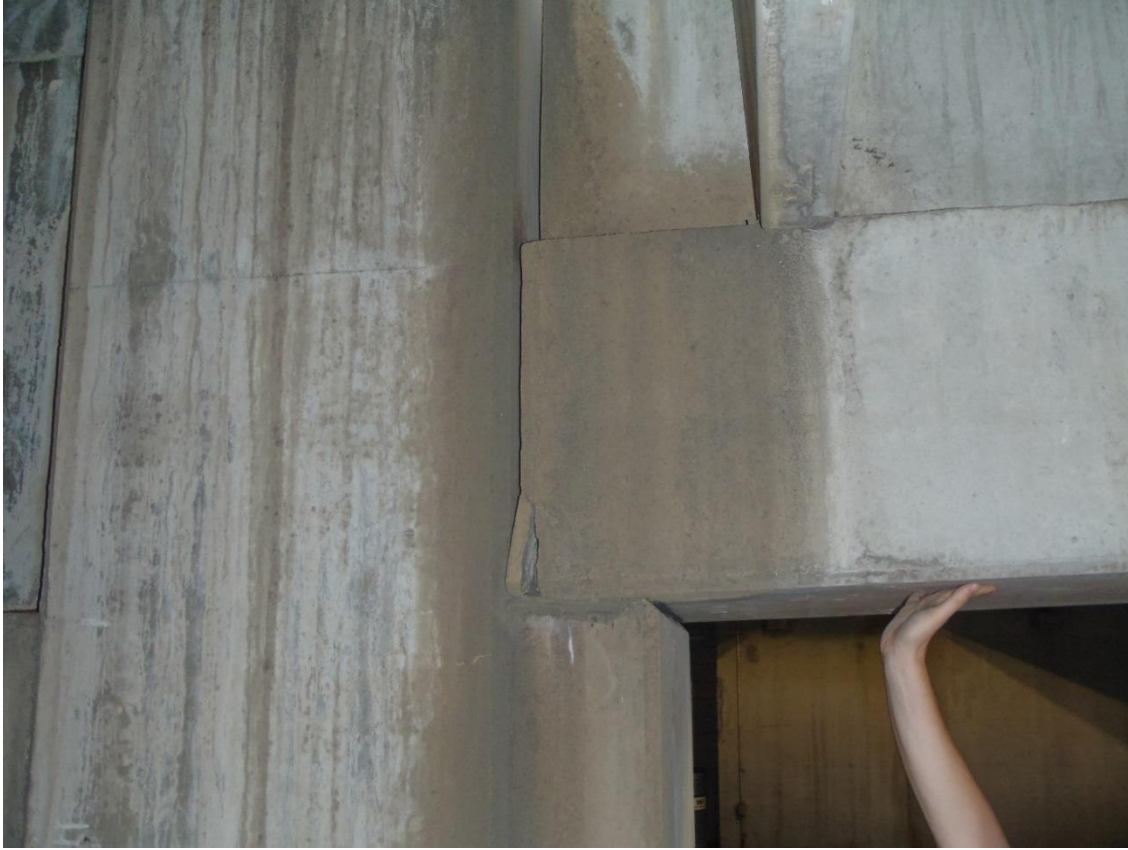
Precast Beam Haunch
