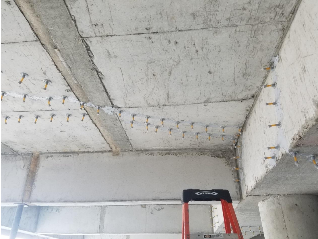
Cracks \geq .035"
