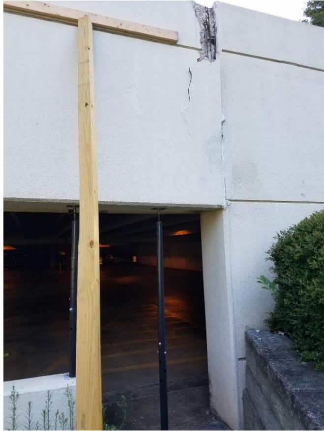
Broken Precast Spandrel Beam
