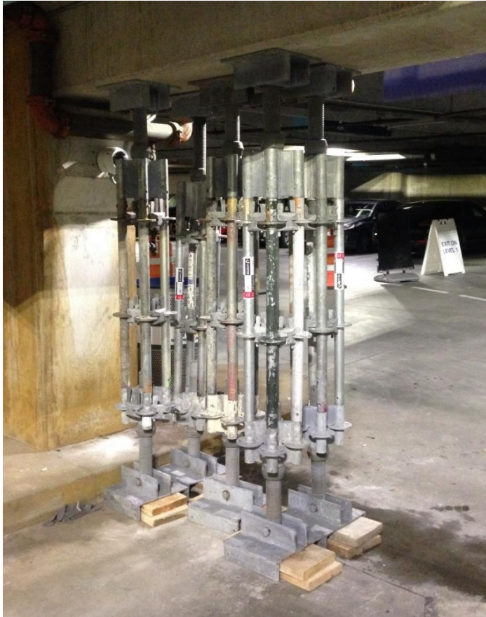
Shoring to Remove Load
