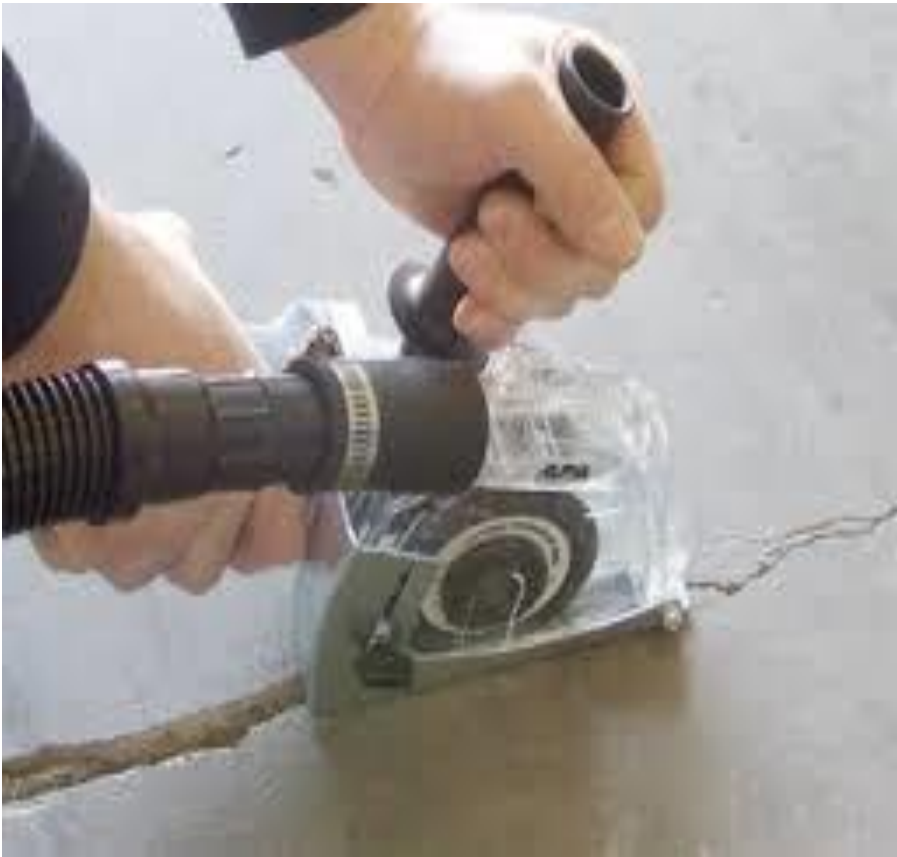
Crack Chasing
