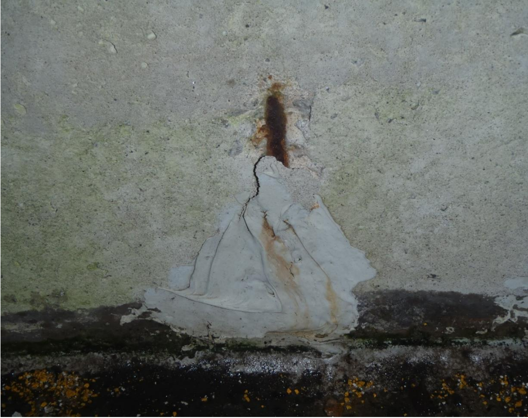
Improper Surface Preparation
