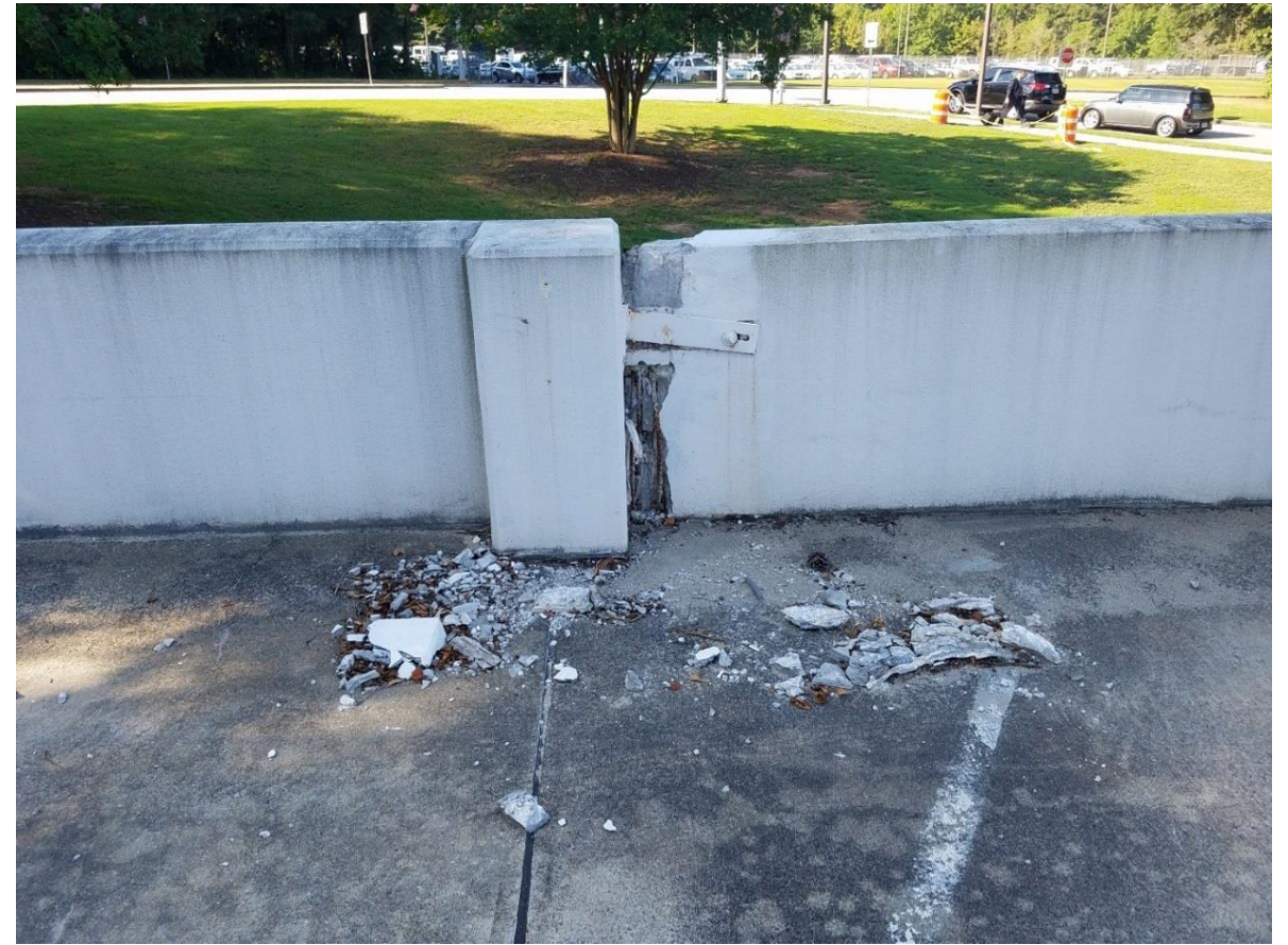
Broken Precast Spandrel Beam
