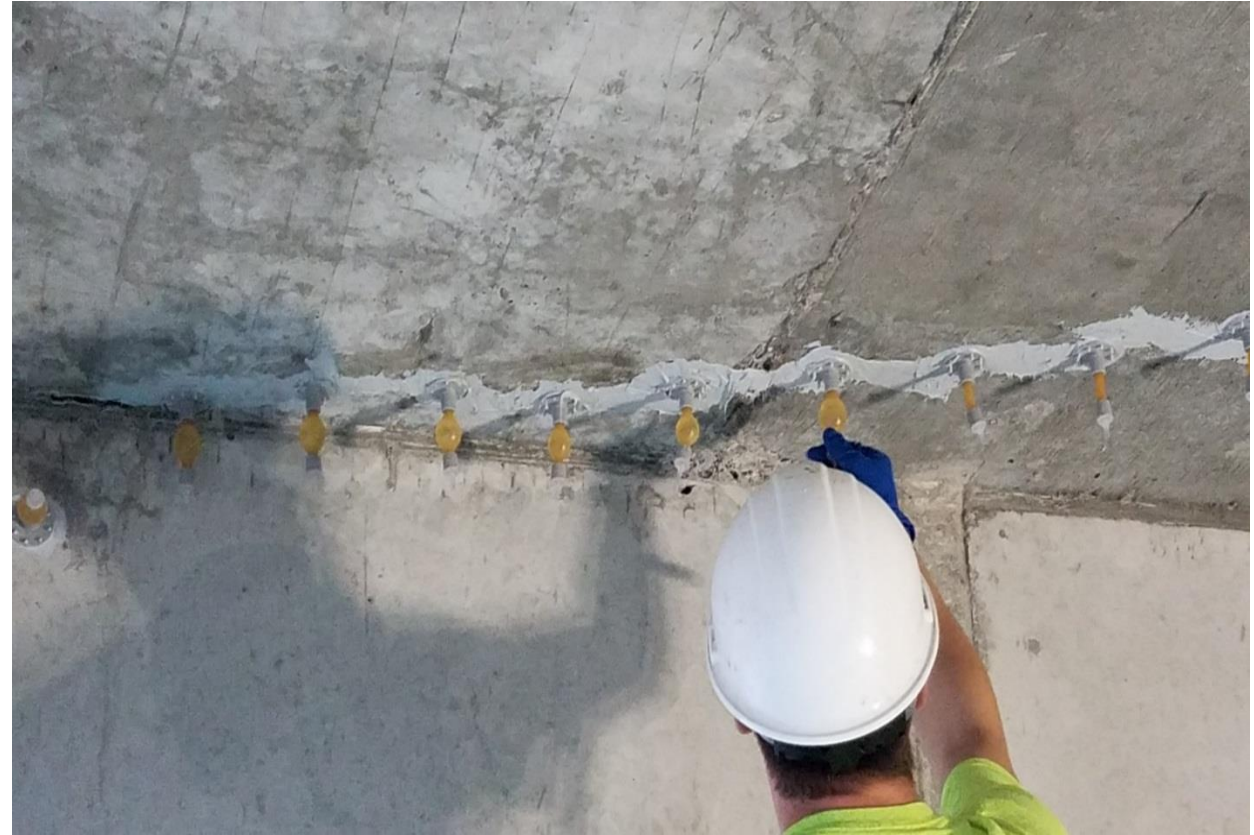
Inflatable Injection Port
