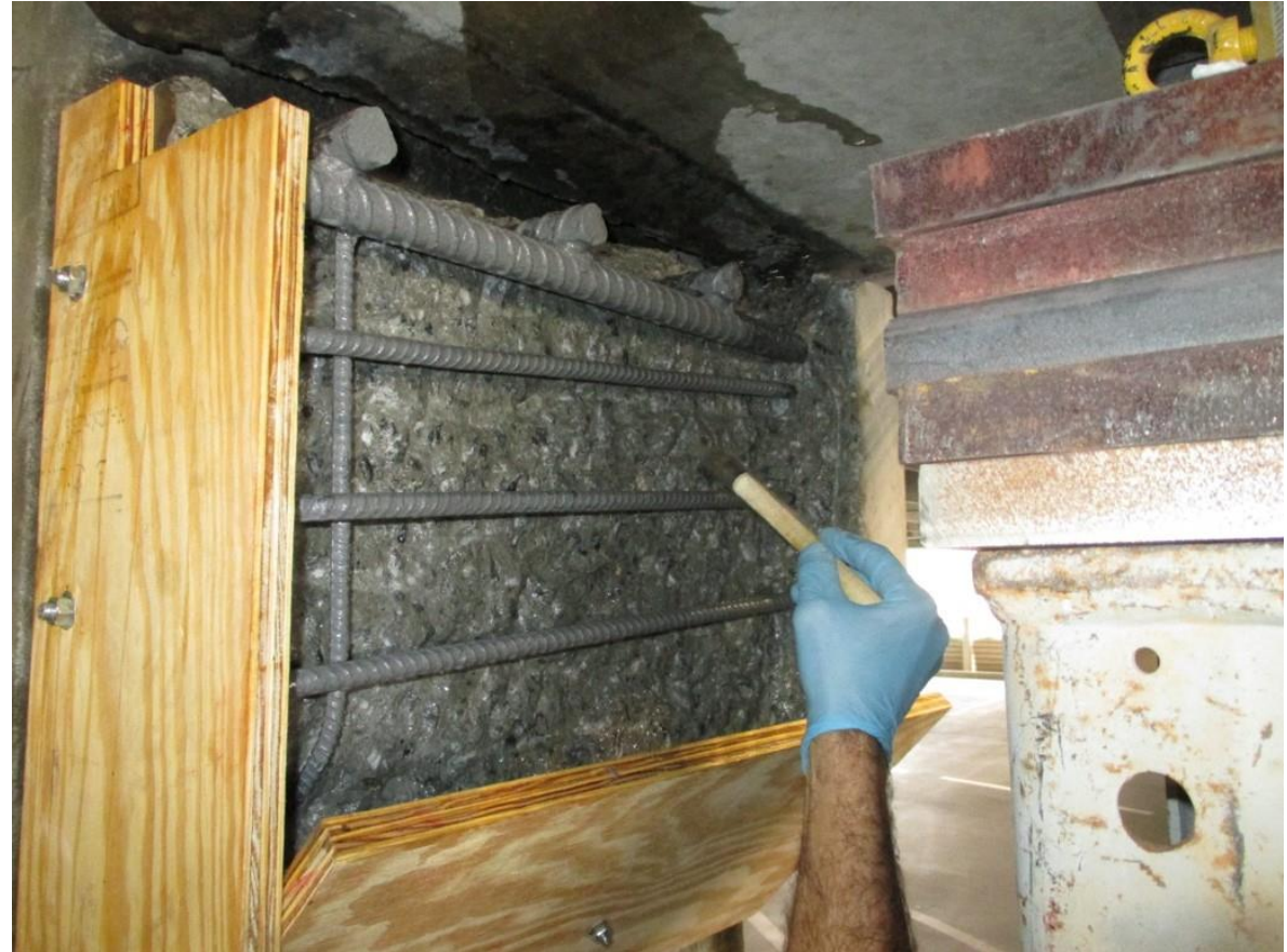
Applying Epoxy Bonding Agent
