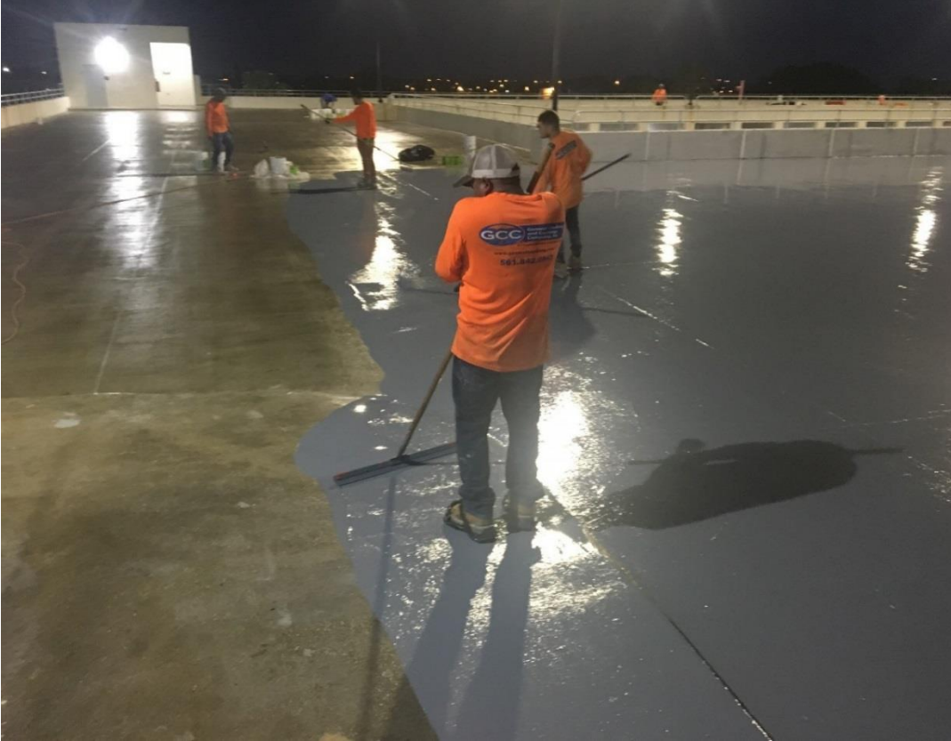
Traffic Bearing Membrane
