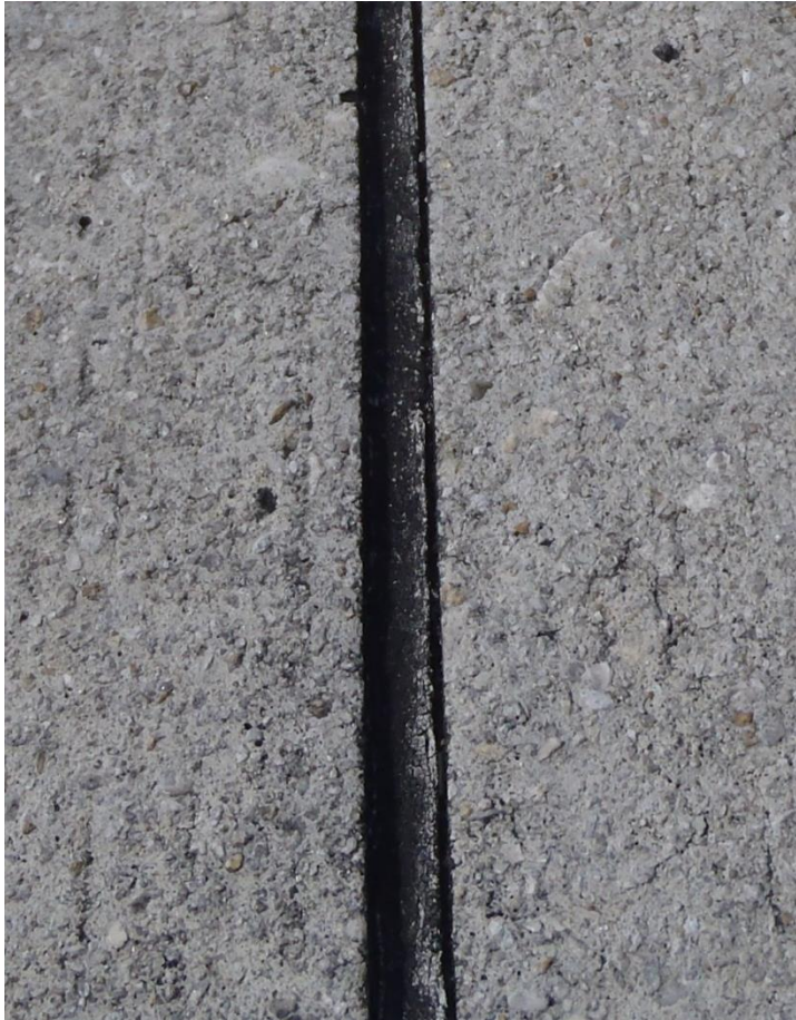
Sealant Failure
