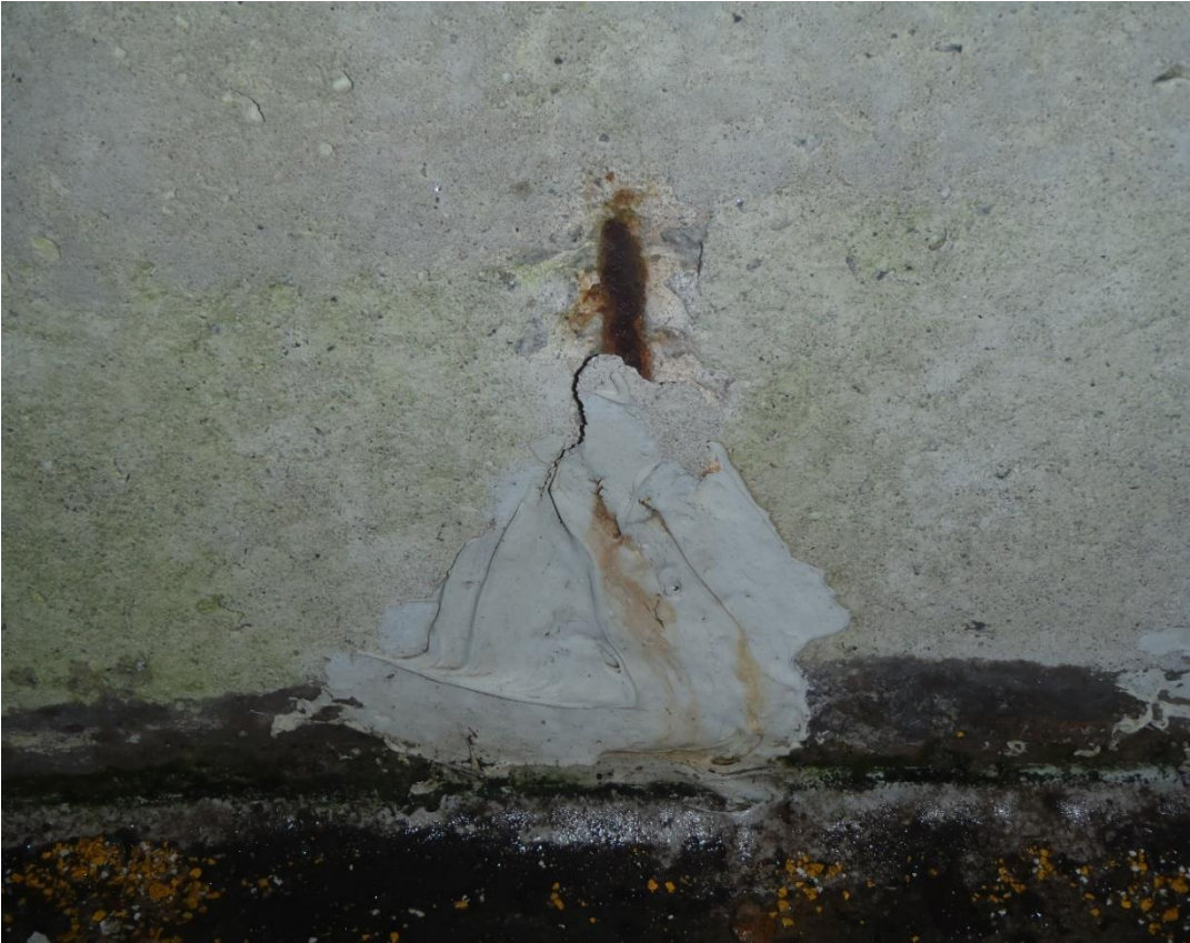
Improper Surface Preparation
