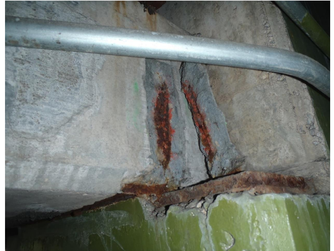
Improper Surface Preparation
