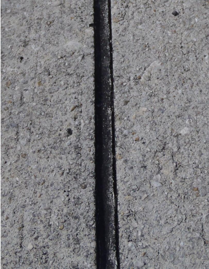
Sealant Failure
