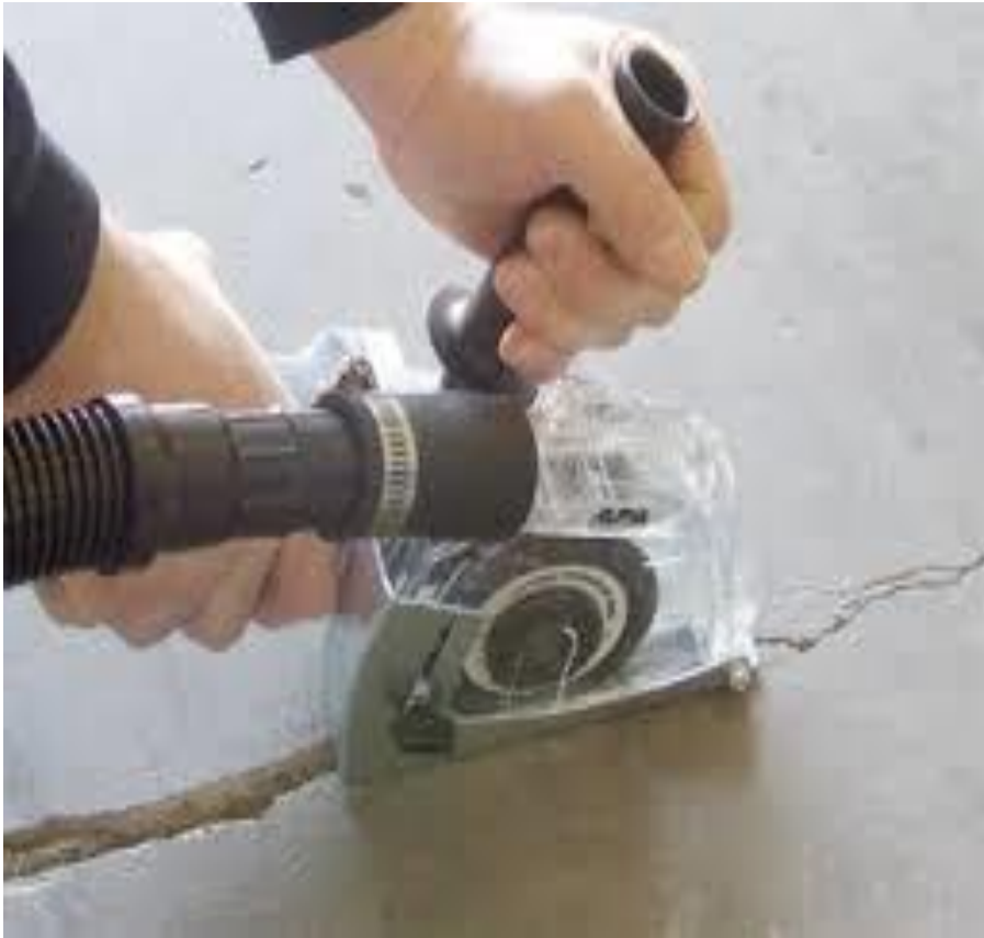
Crack Chasing
