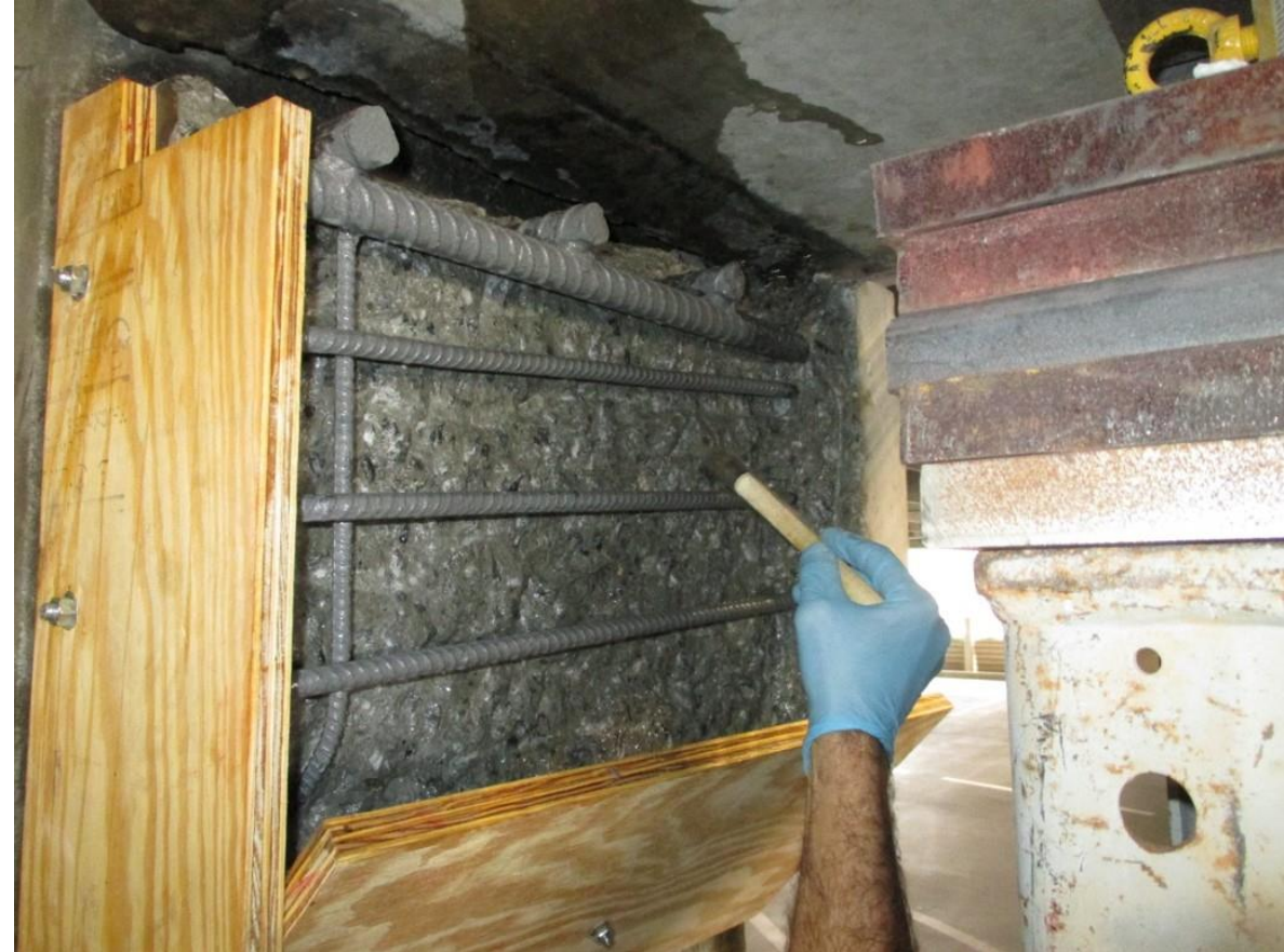
Applying Epoxy Bonding Agent
