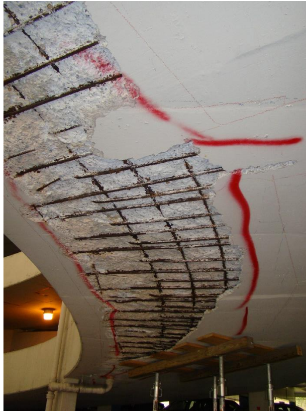
Delamination
