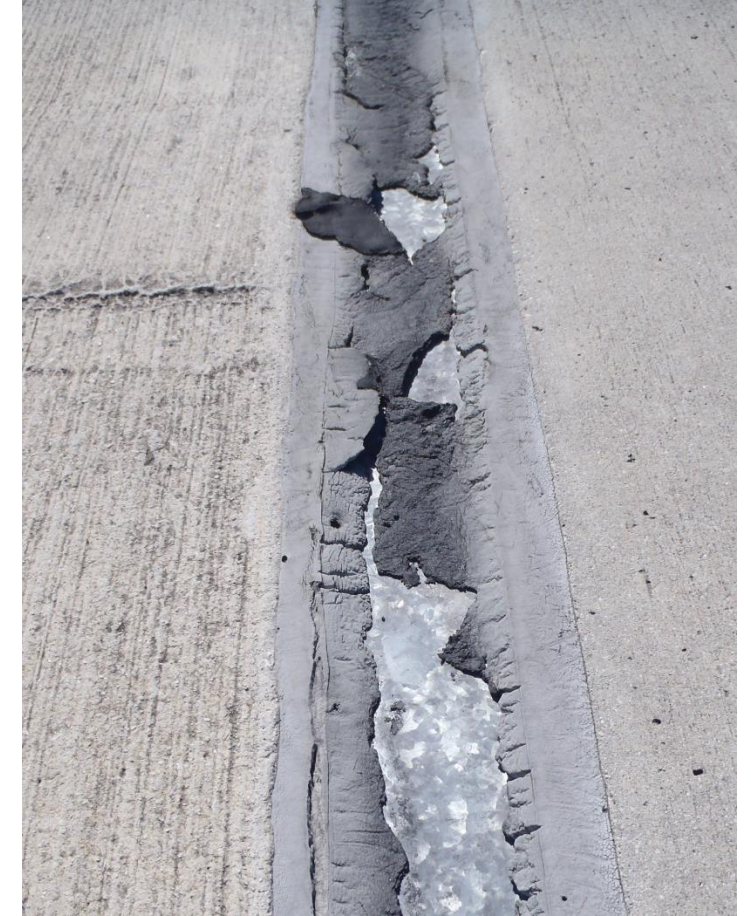
Expansion Joint Failure
