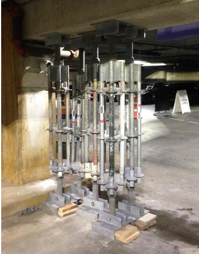
Shoring to Remove Load
