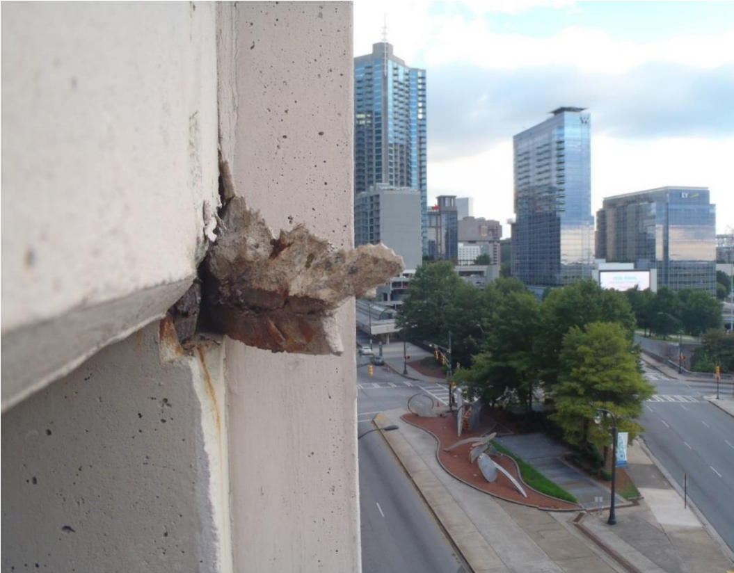
Spall Over Sidewalk
