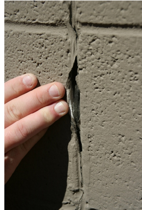
Failed Sealant
