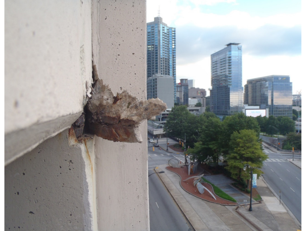
Concrete Spalls
