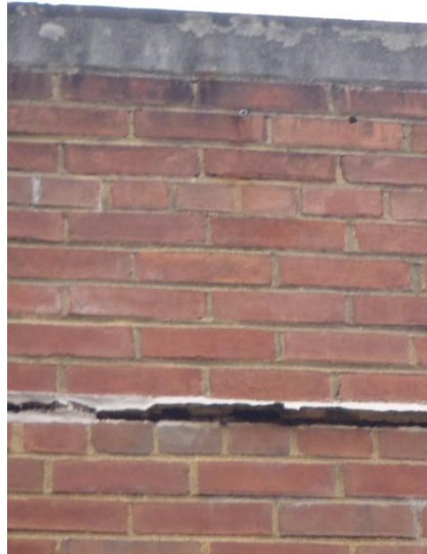
Bond Break at Roof Line
