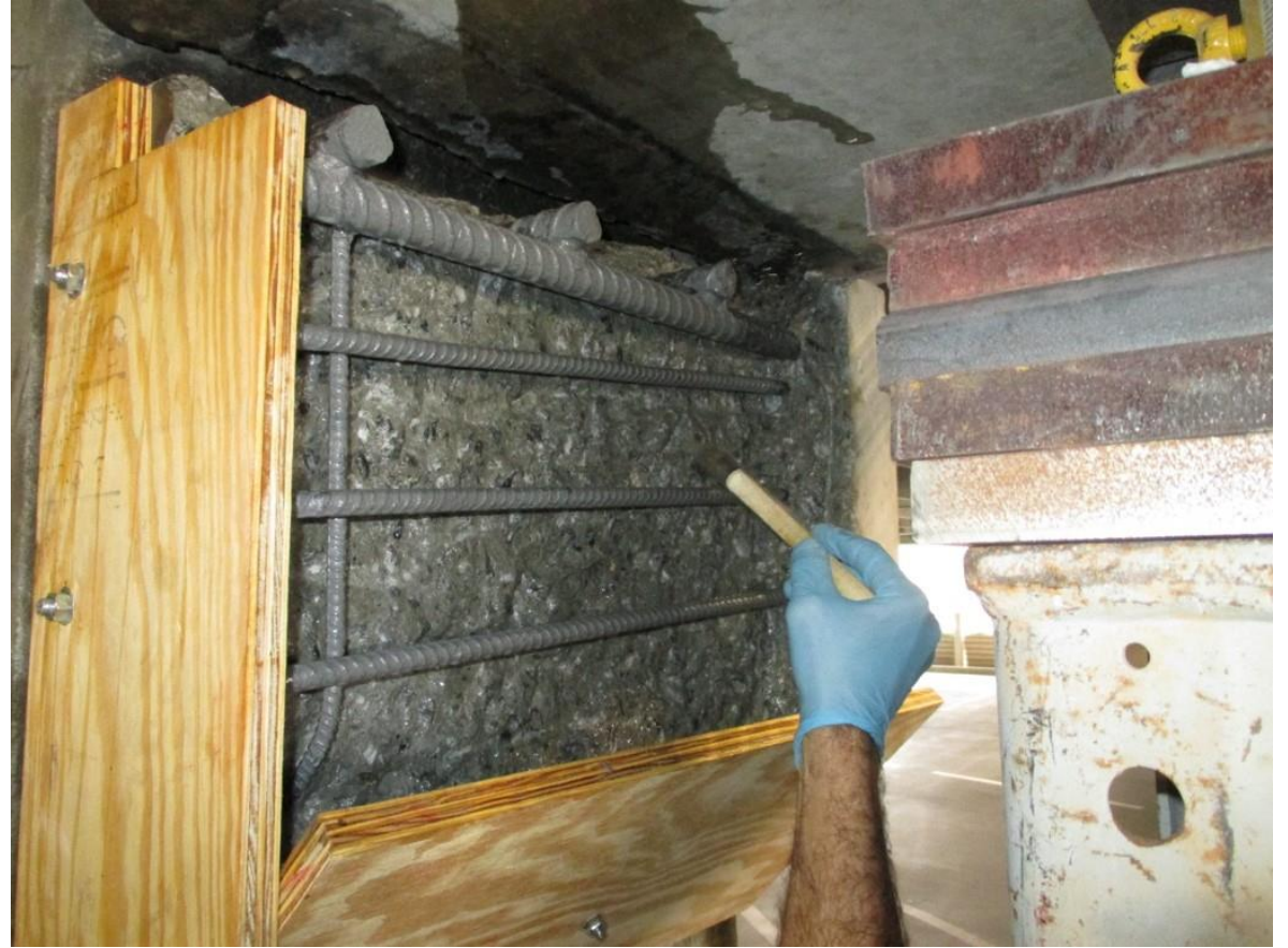
Applying Epoxy Bonding Agent
