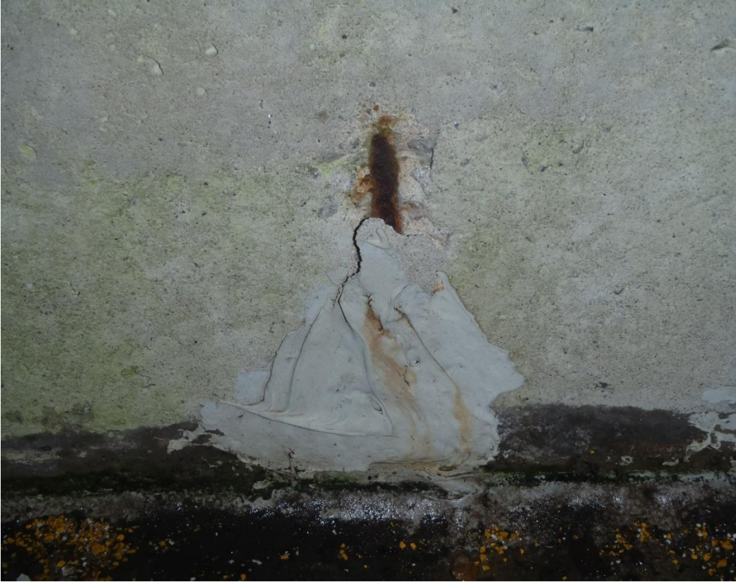
Improper Surface Preparation
