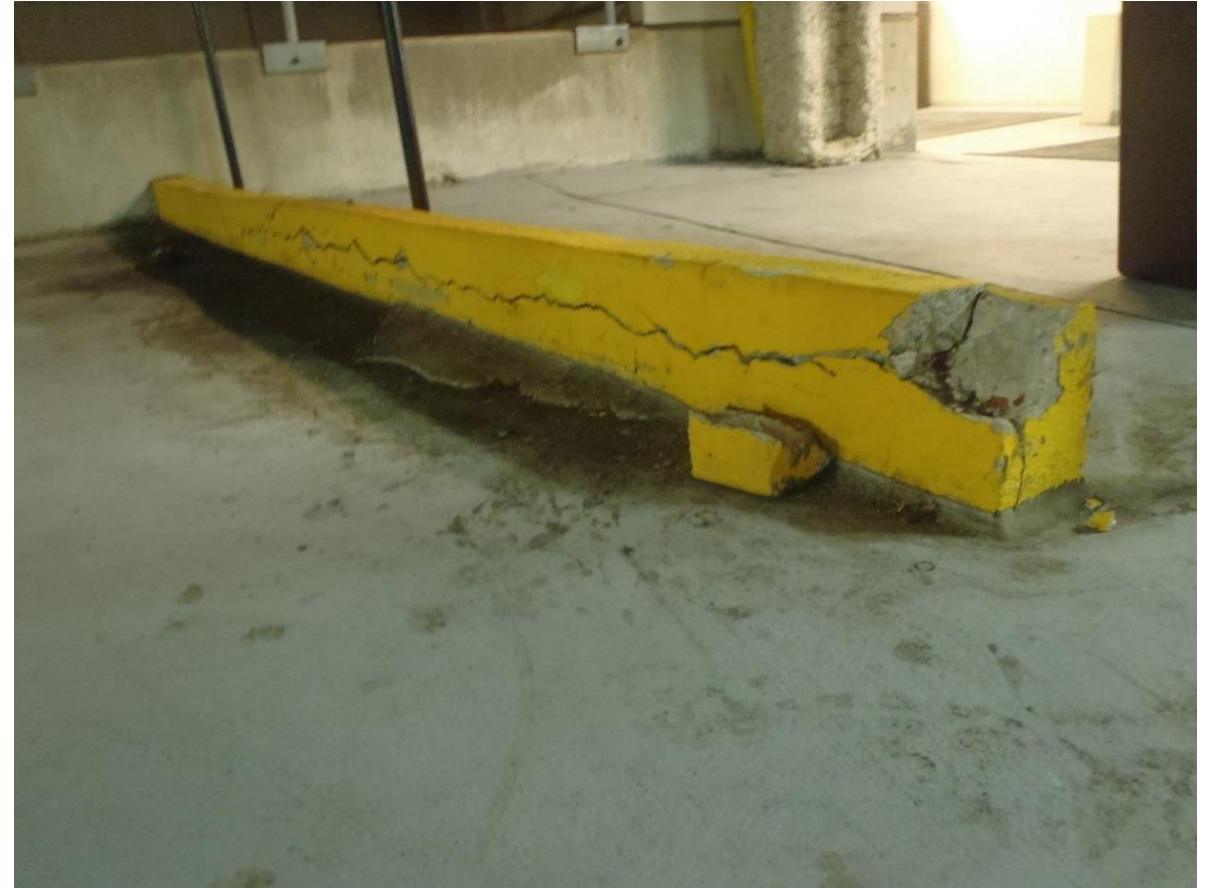
Broken Precast Spandrel Beam
