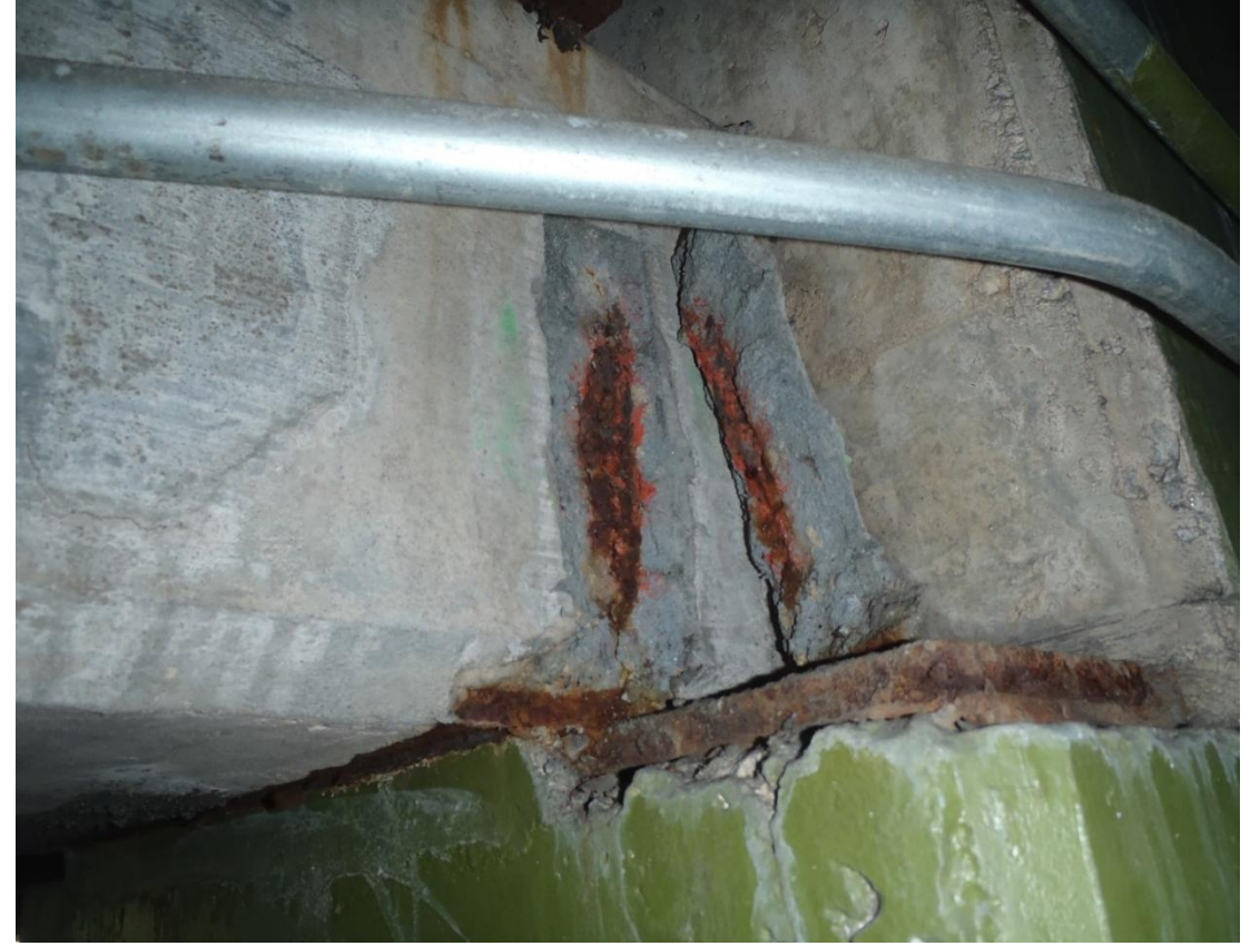
Improper Surface Preparation
