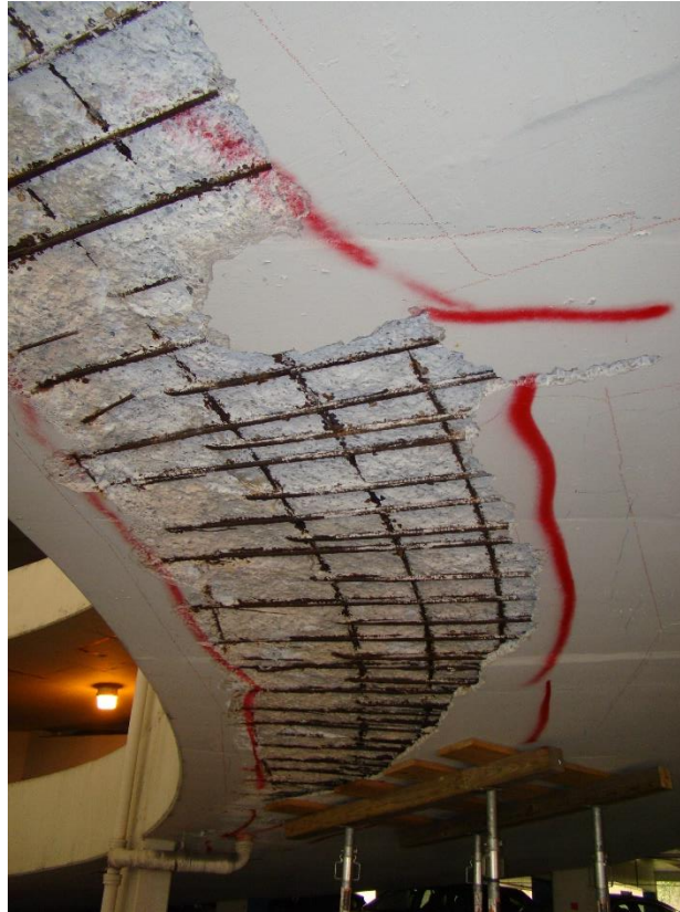
Delamination
