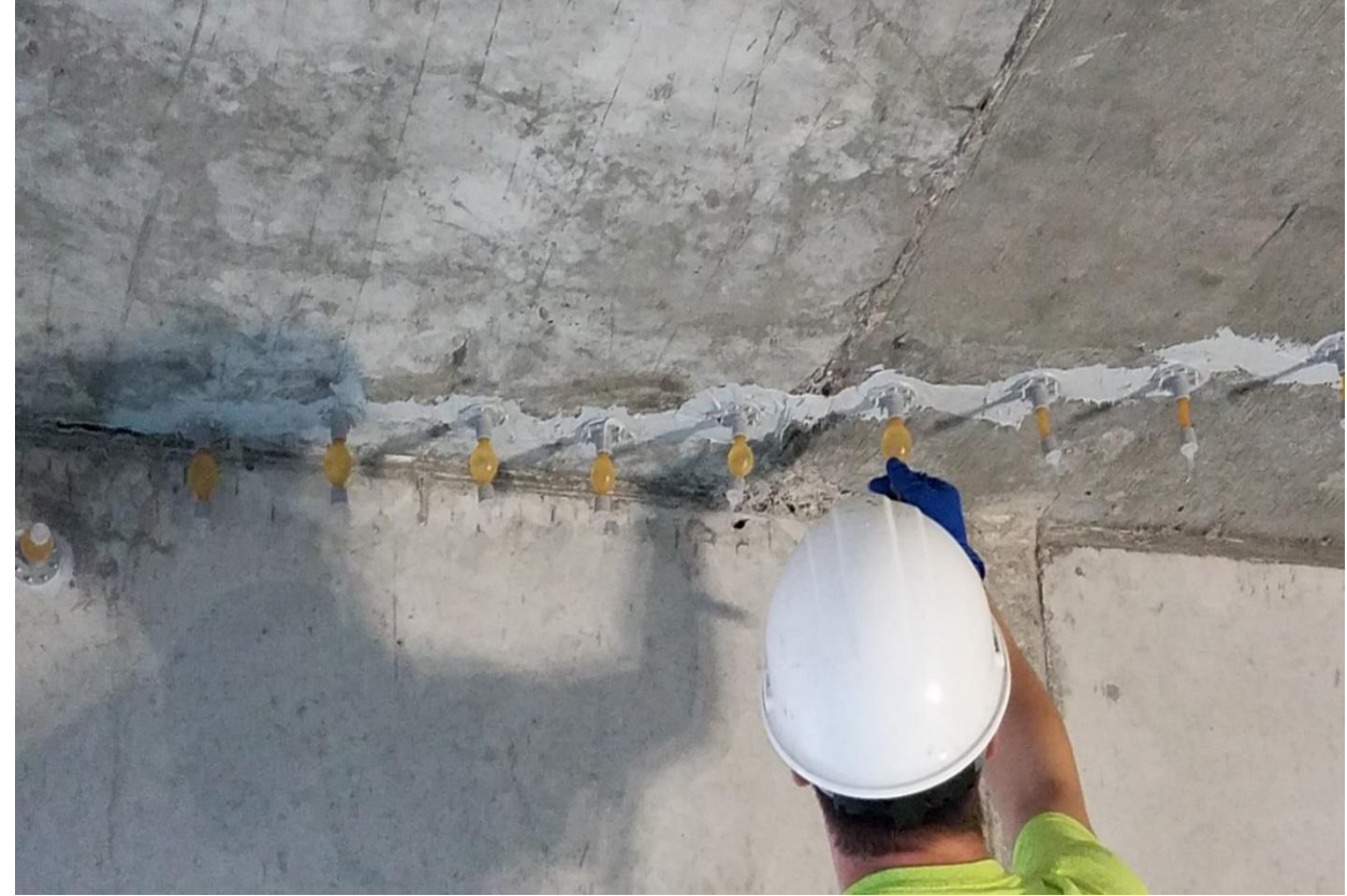
Inflatable Injection Port
