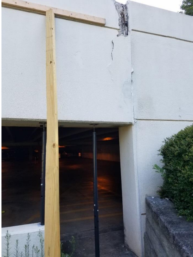
Broken Precast Spandrel Beam
