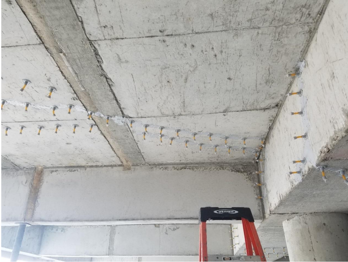
Cracks \geq .035''
