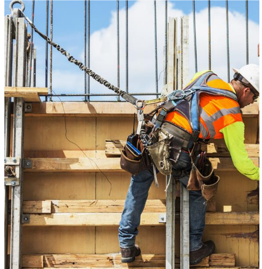
Fall Arrest – 6 Ft. Shock Absorbing Lanyard
