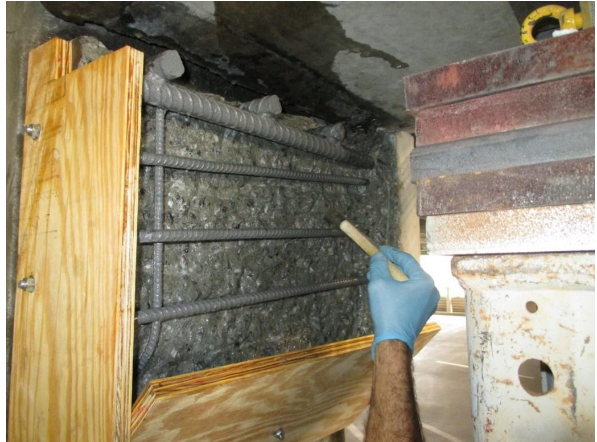
Applying Epoxy Bonding Agent
