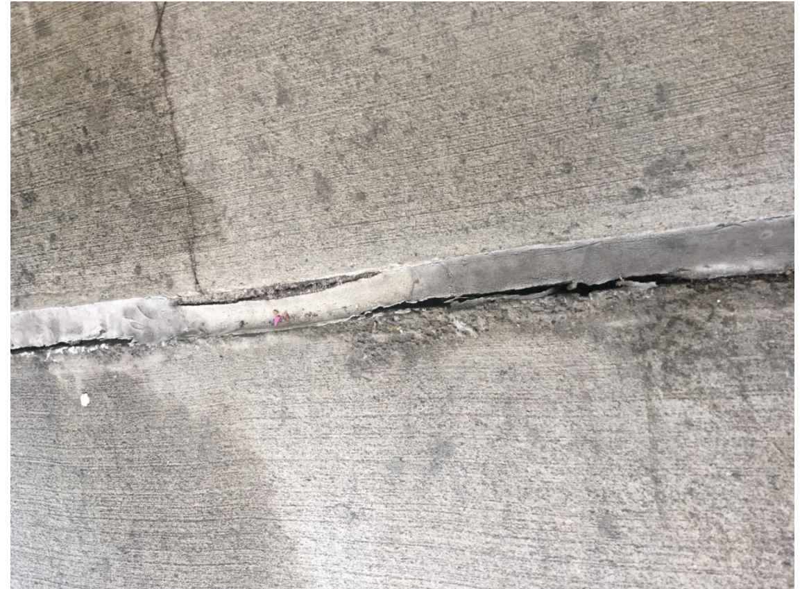
Adhesive Failure
