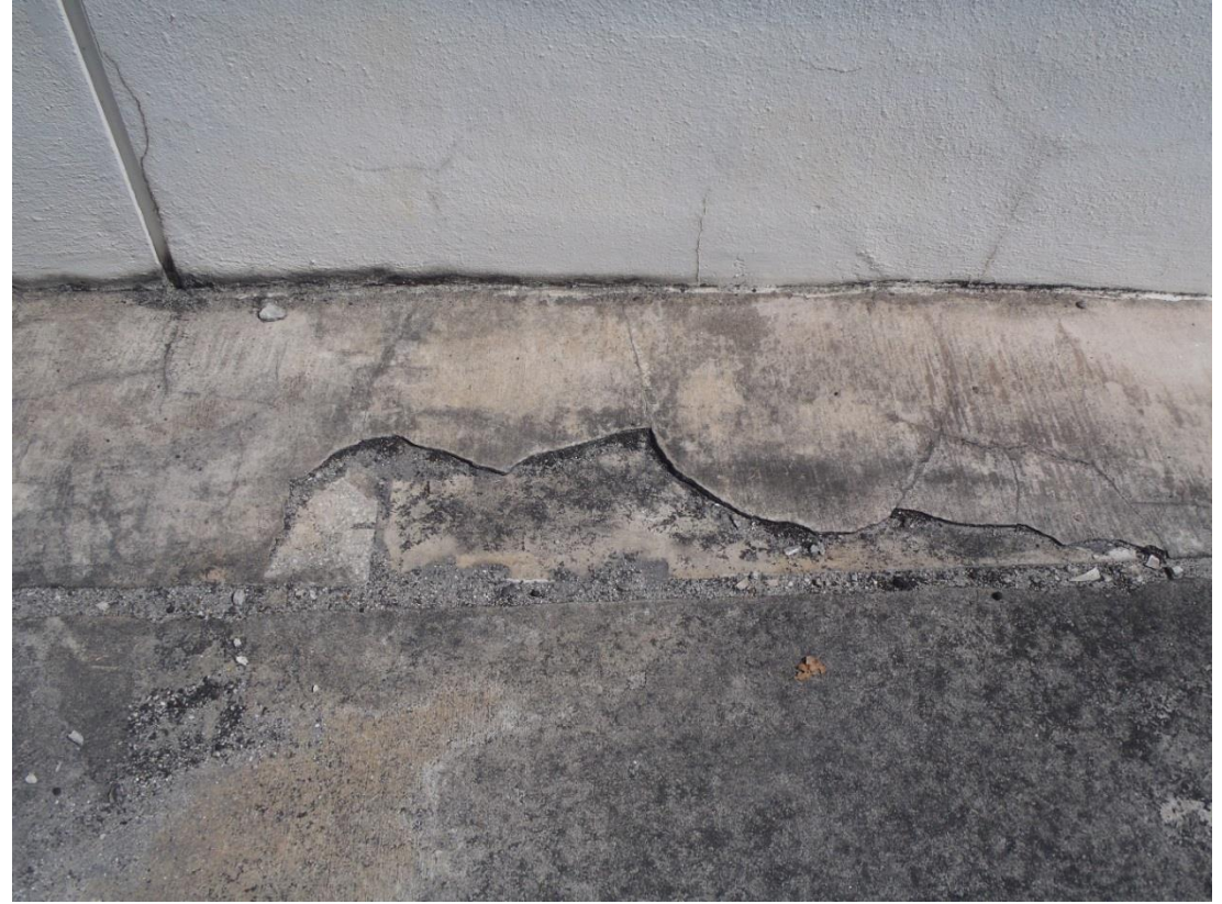
Topping Delamination
