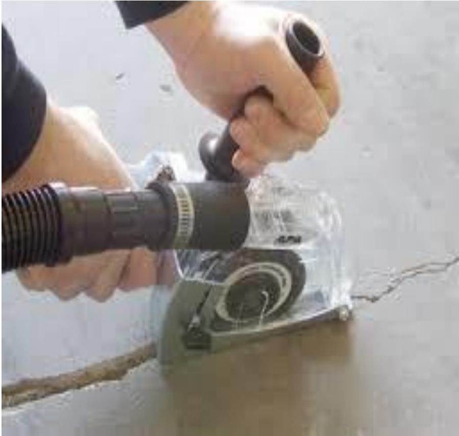
Crack Chasing
