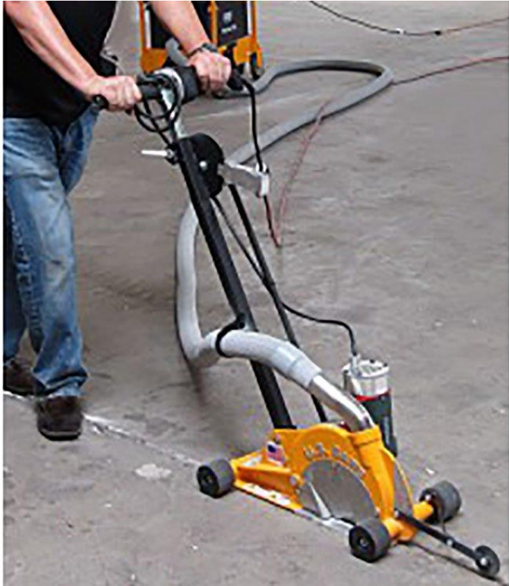
Grinding Joint
