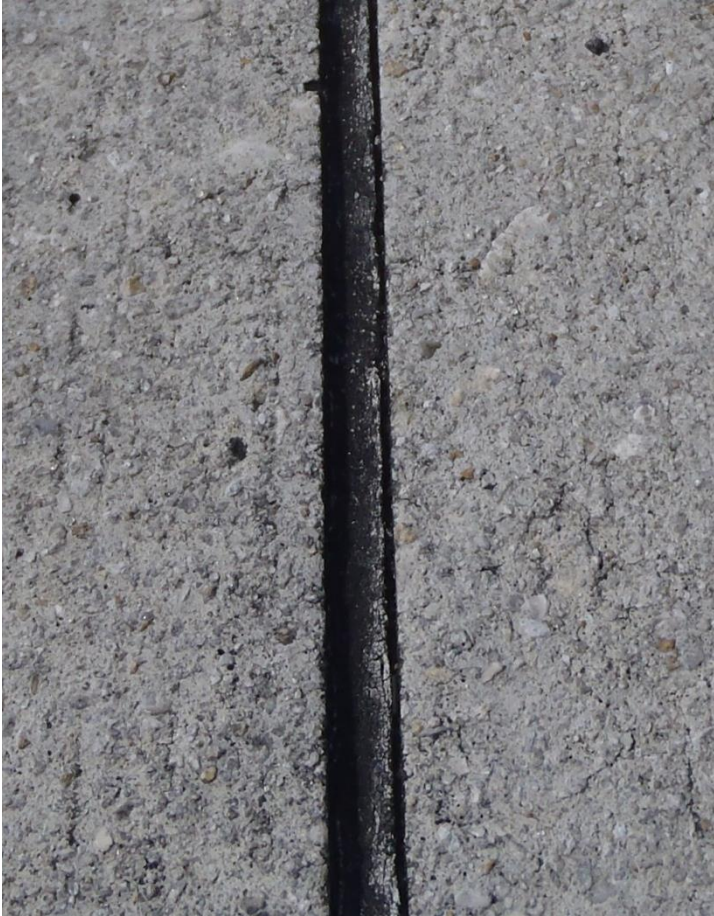
Sealant Failure
