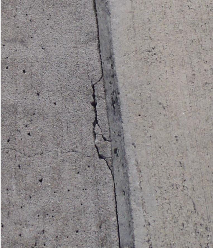
Substrate Failure
