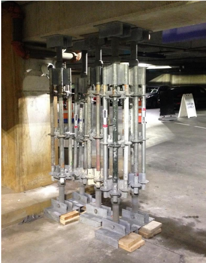
Shoring to Remove Load
