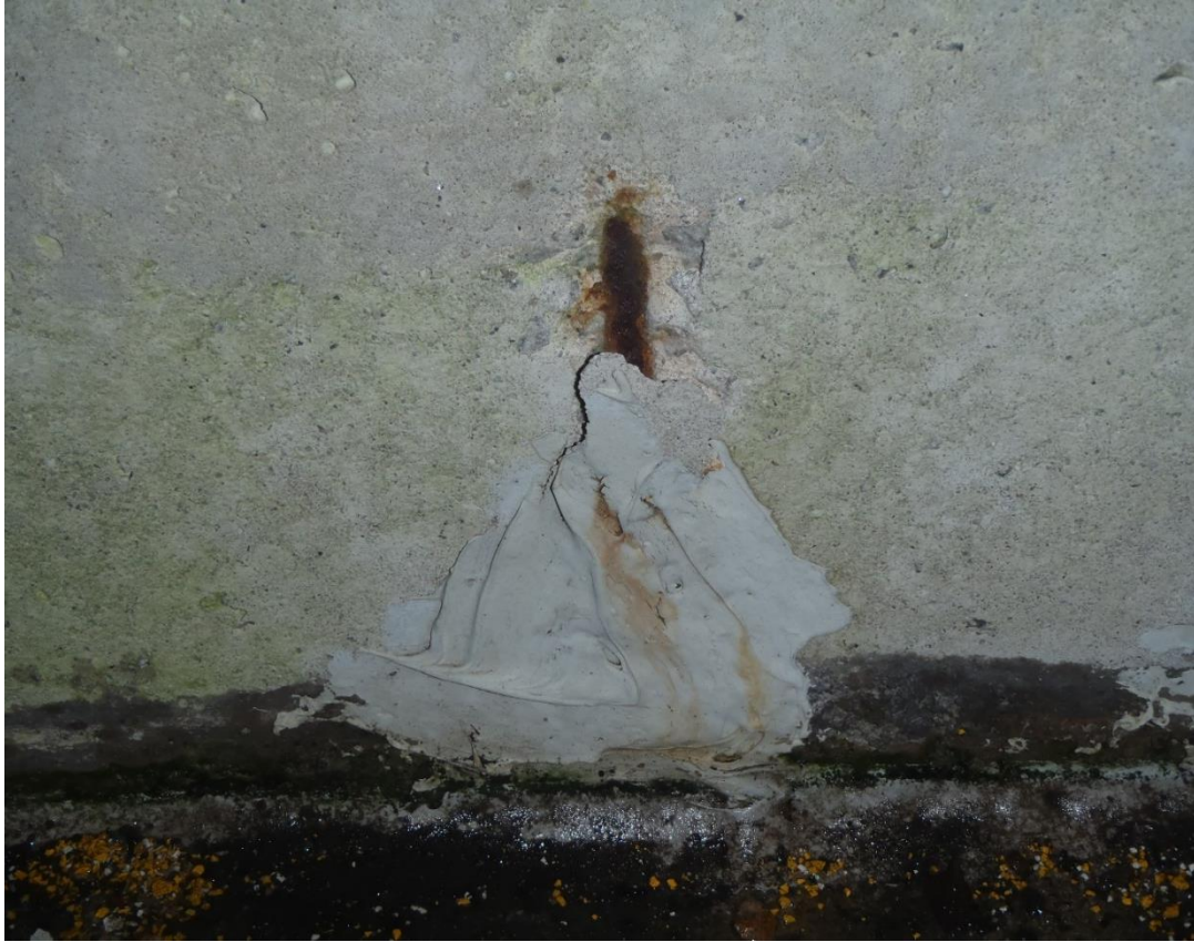
Improper Surface Preparation
