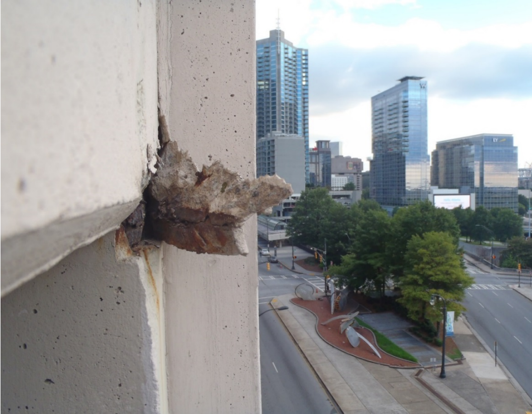
Spall Over Sidewalk
