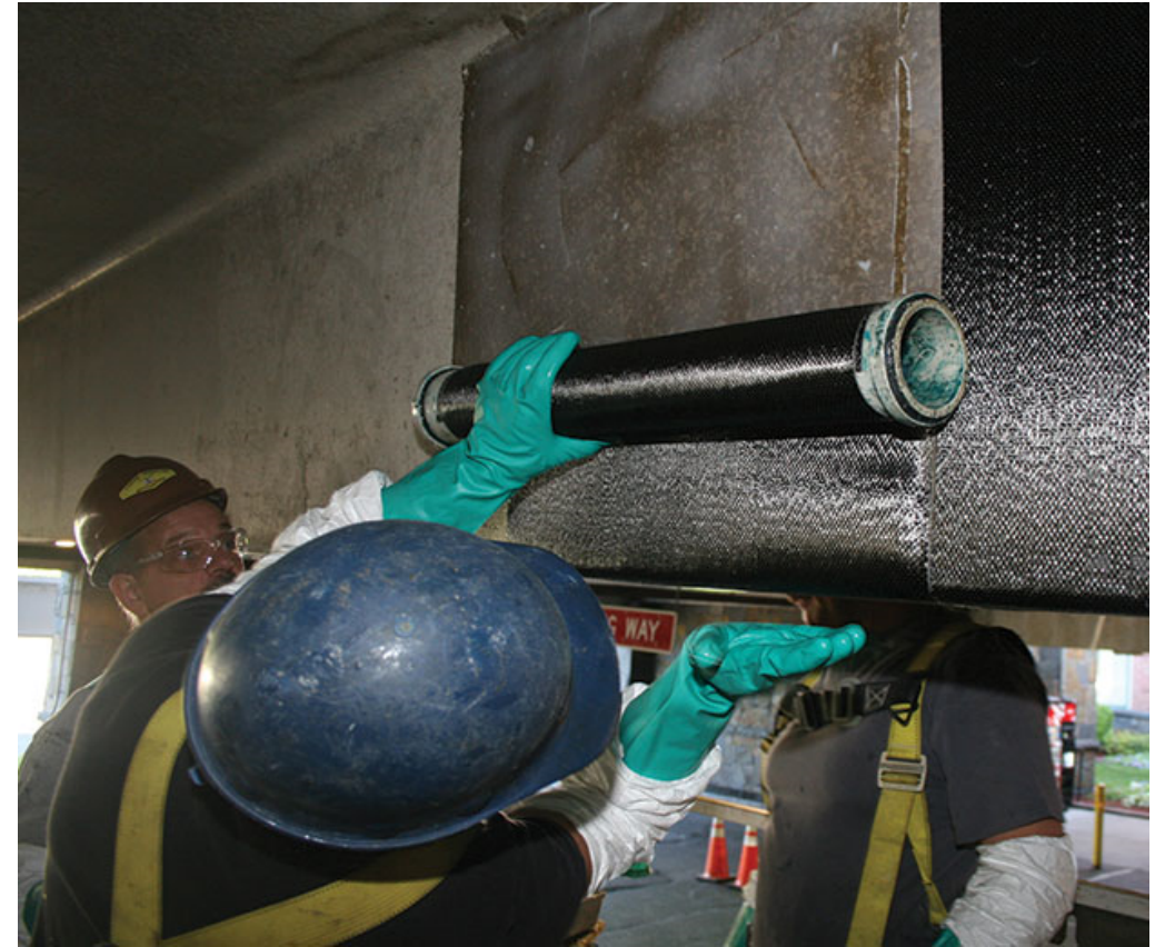
CFRP Repair
