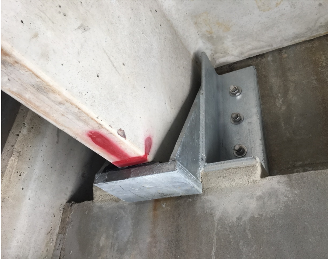
Steel Seat Repair
