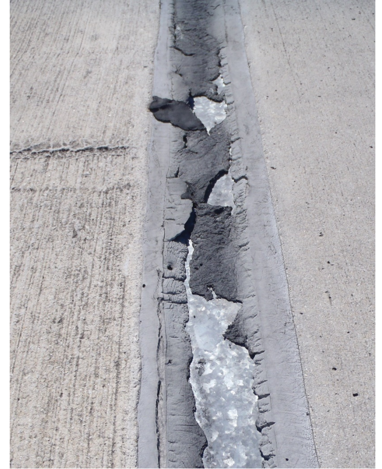
Expansion Joint Failure
