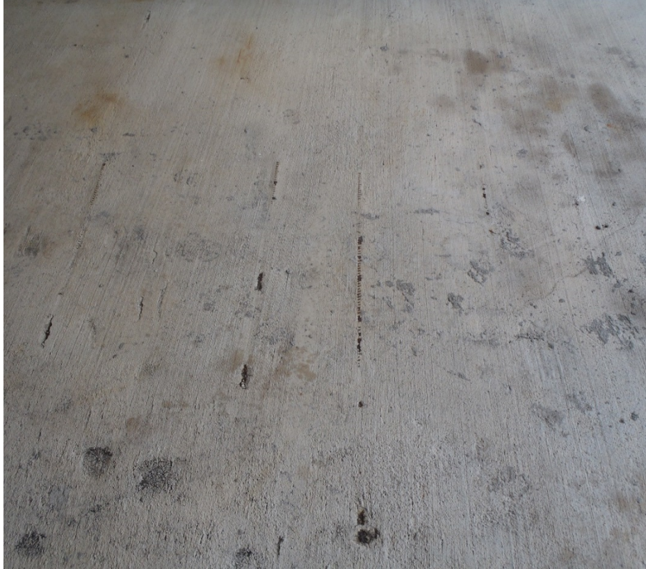
Exposed Reinforcing Steel
