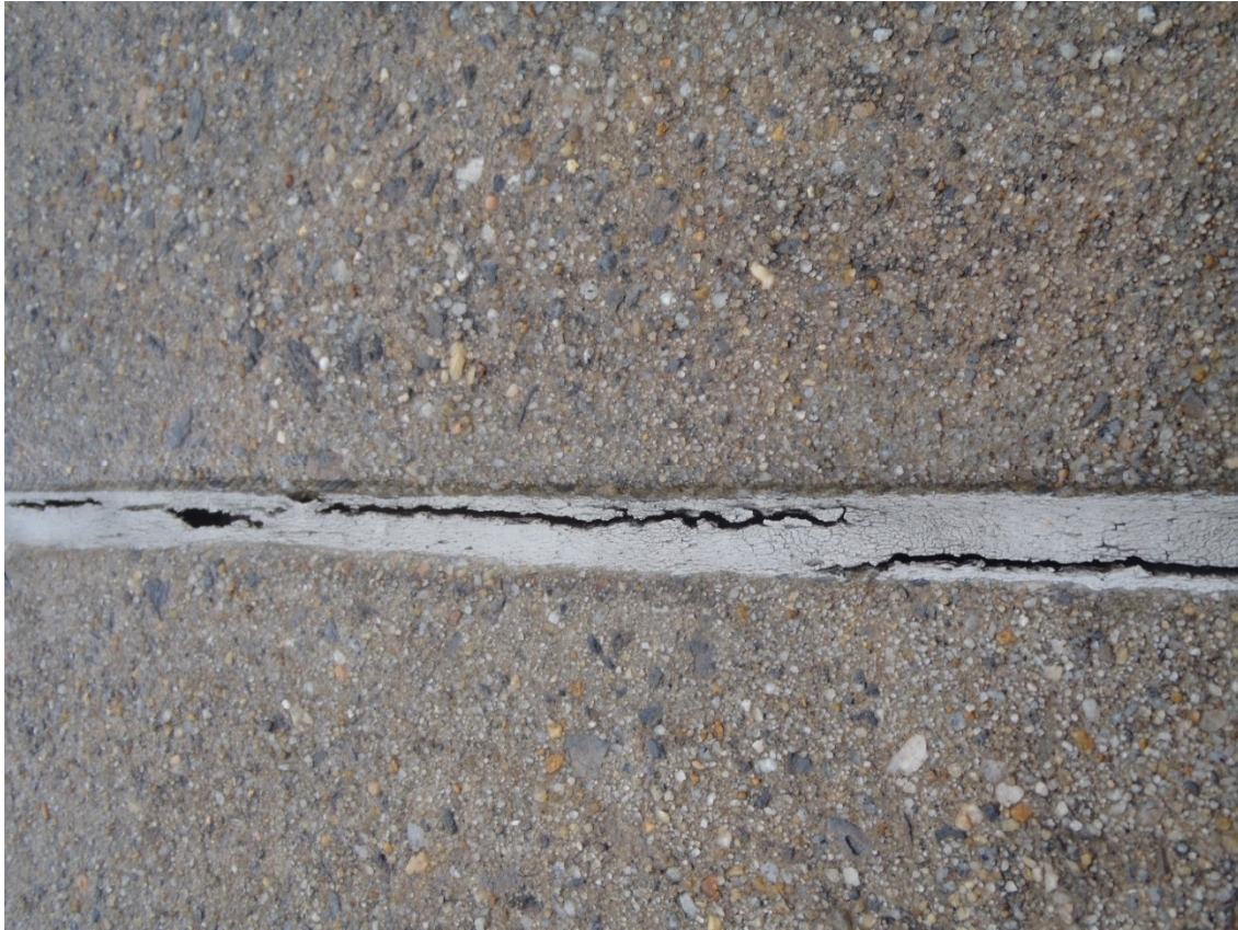
Cohesive Failure/Aged & Weathered
