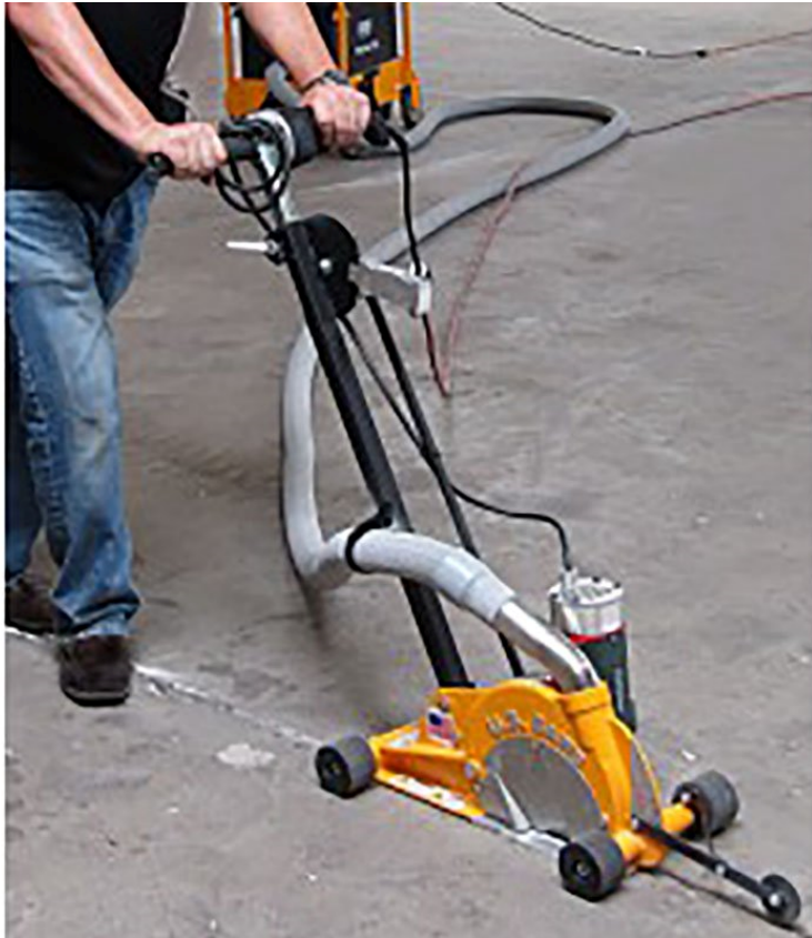
Grinding Joint
