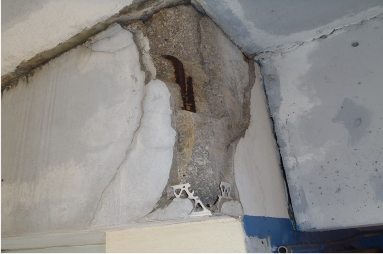
Rust Expansion & Spalling
