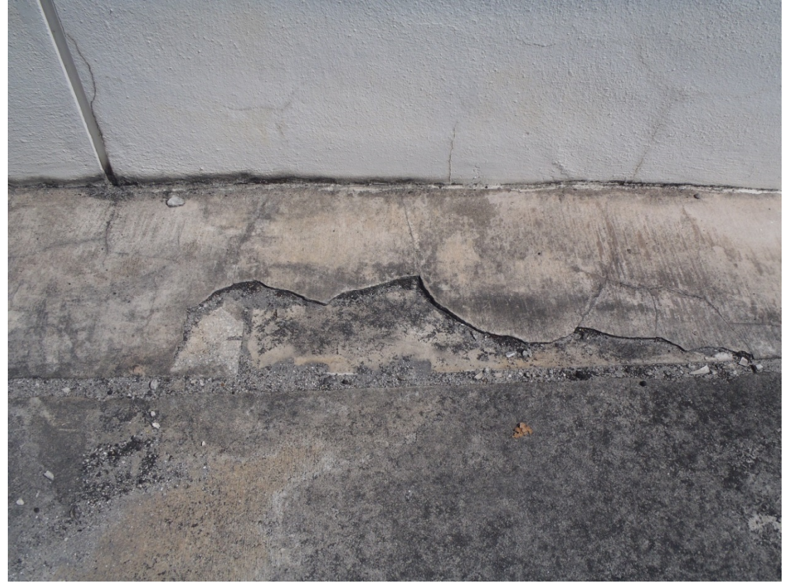
Topping Delamination
