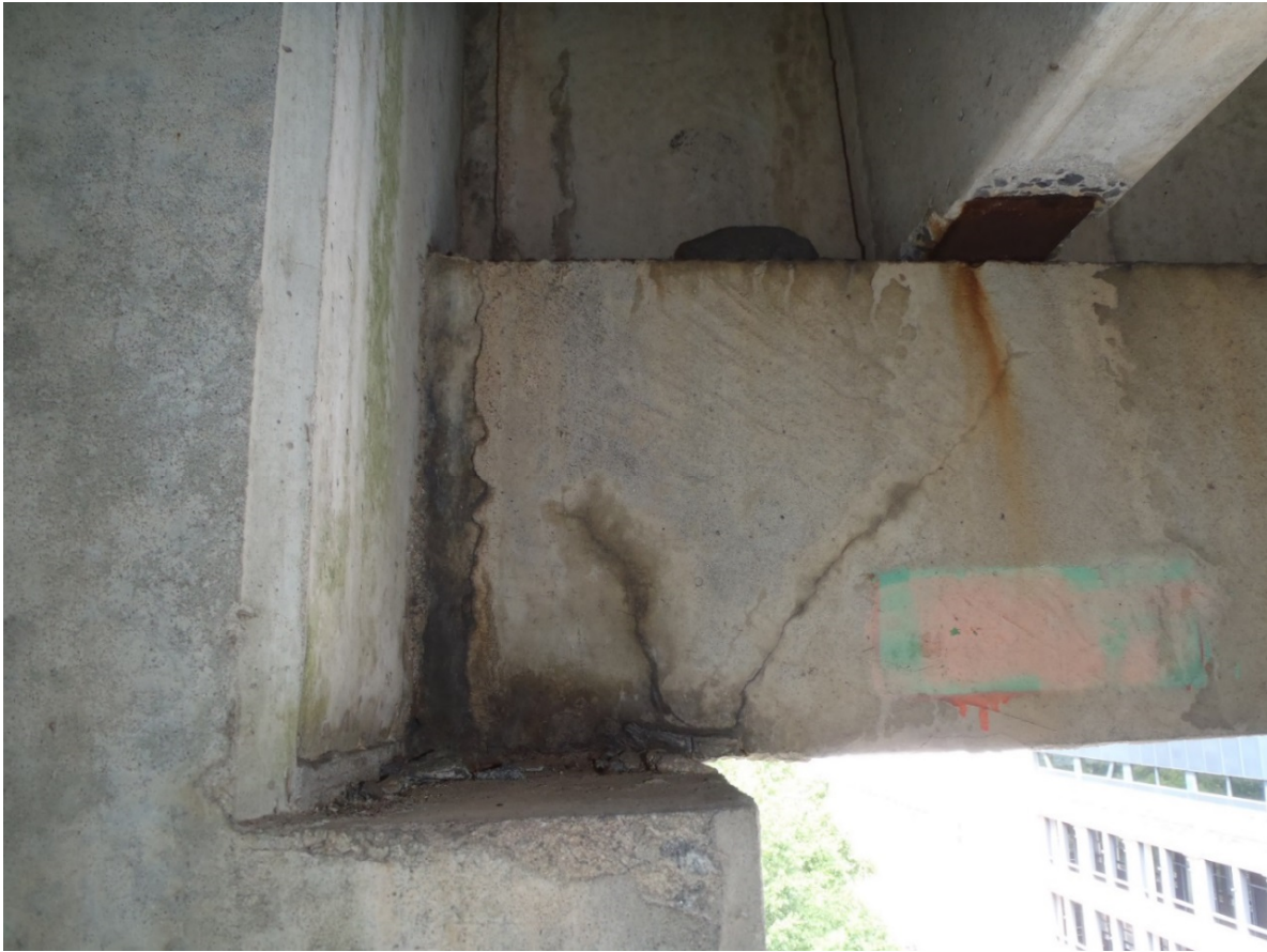
Shear Crack
