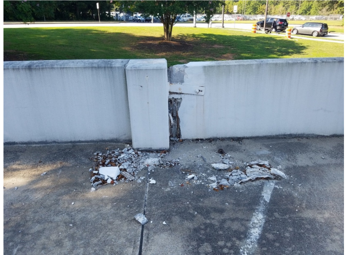
Broken Precast Spandrel Beam
