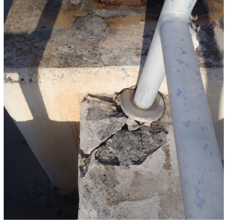
Broken End Connection
