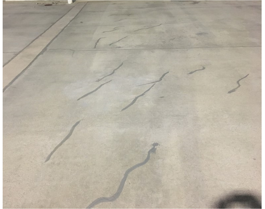
Crack Sealant
