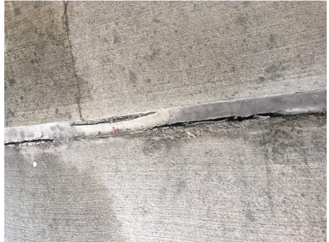
Adhesive Failure
