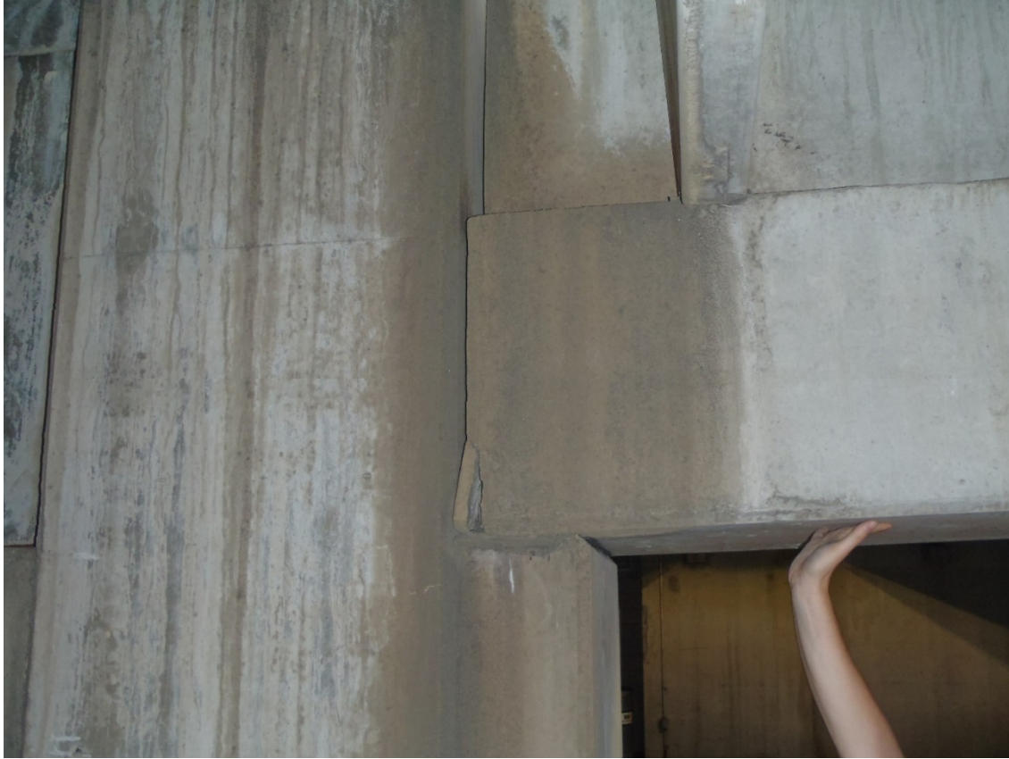
Precast Beam Haunch
