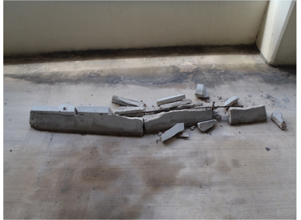
Broken Wheel Stop
