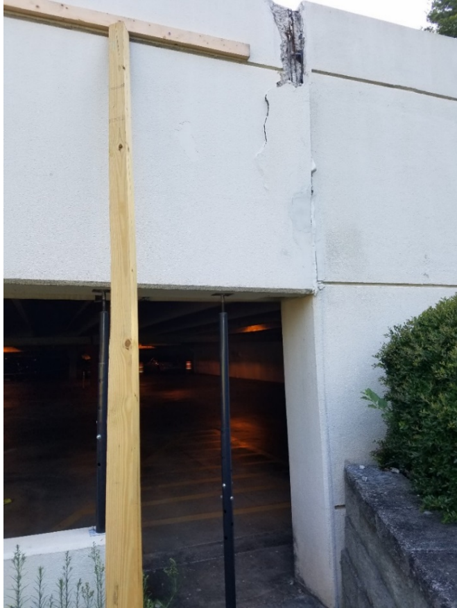
Broken Precast Spandrel Beam
