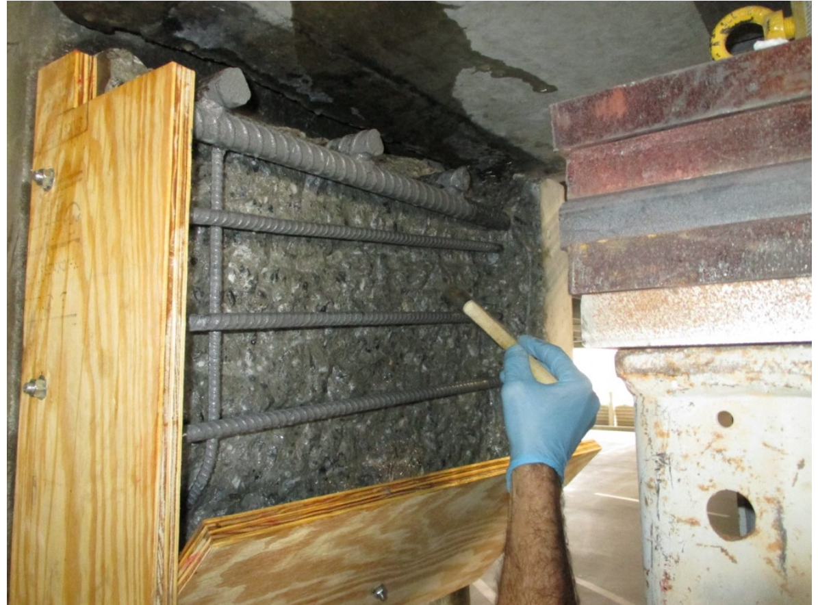
Applying Epoxy Bonding Agent
