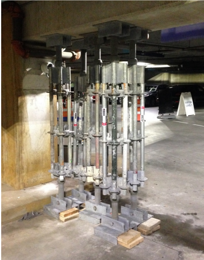
Shoring to Remove Load
