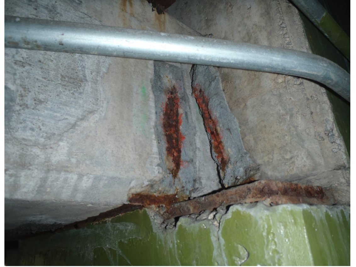
Improper Surface Preparation
