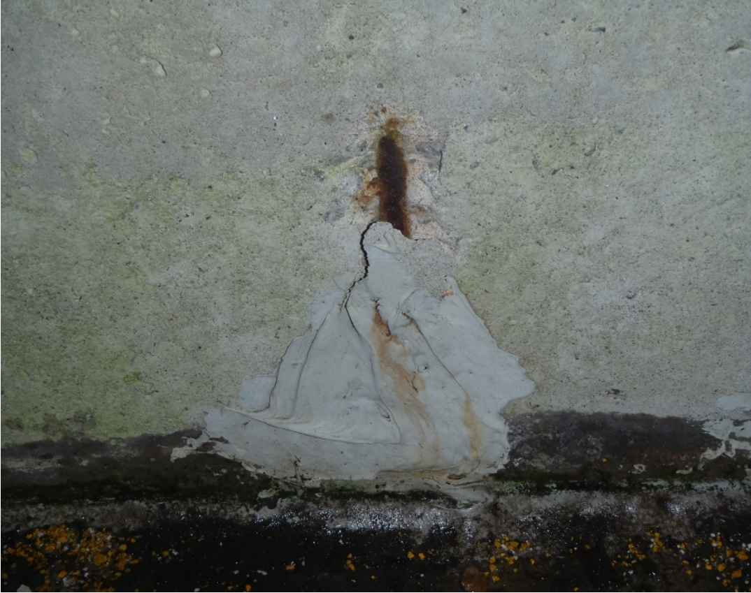
Improper Surface Preparation
