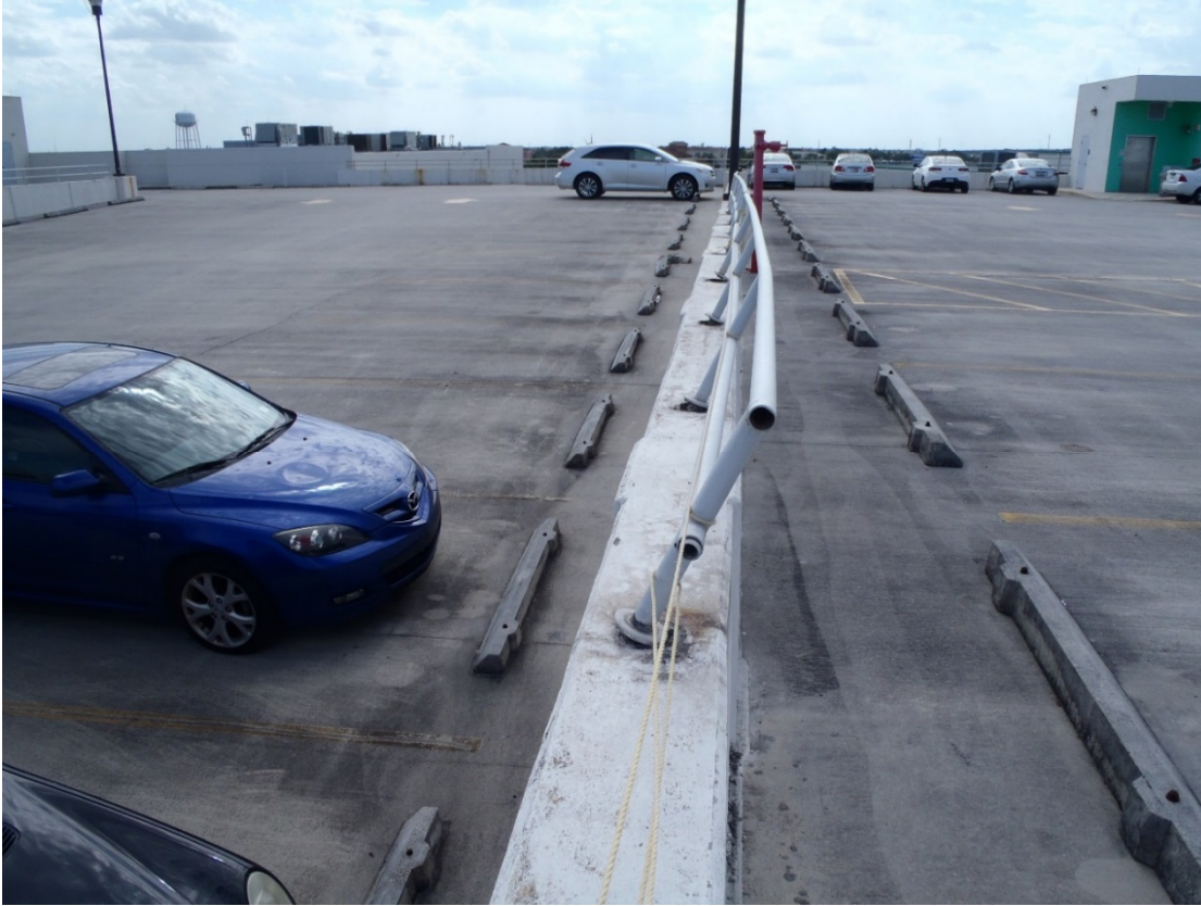
Failed Guardrail
