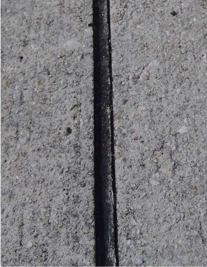
Sealant Failure
