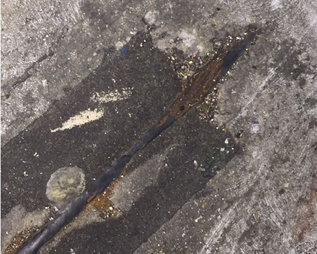
Exposed Post Tensioning (PT)
