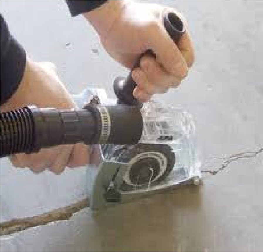
Crack Chasing
