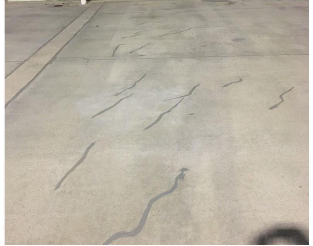
Crack Sealant
