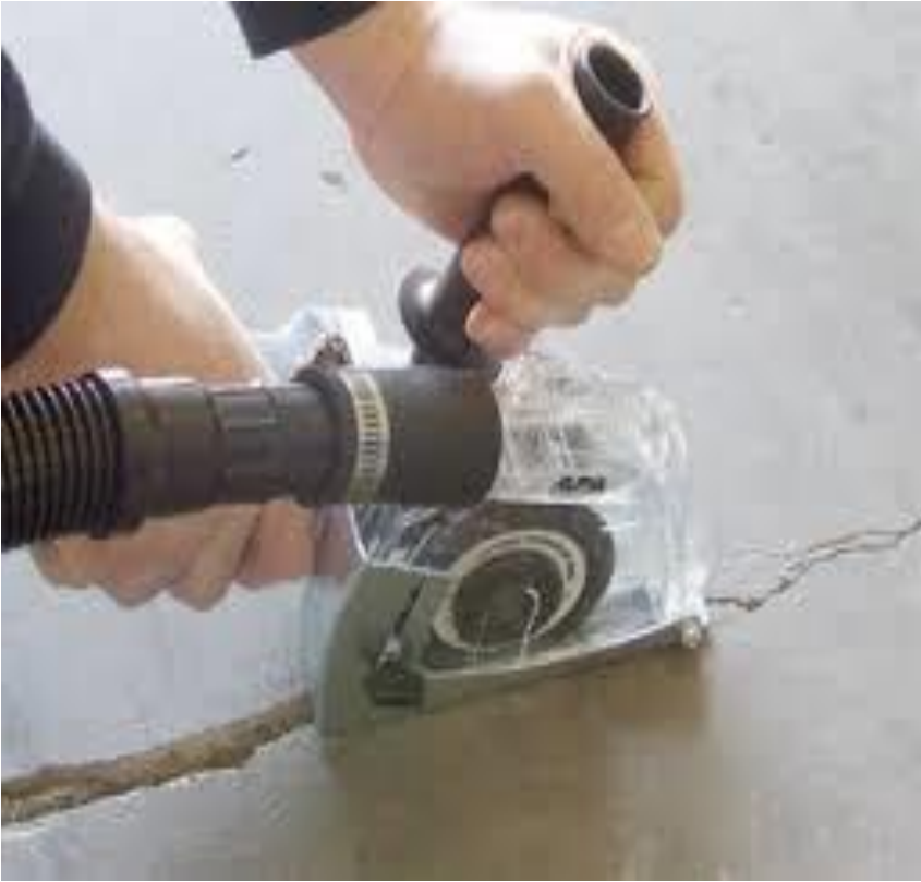
Crack Chasing
