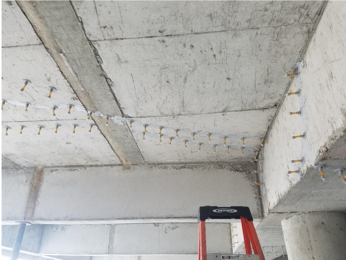
Cracks \geq .035"
