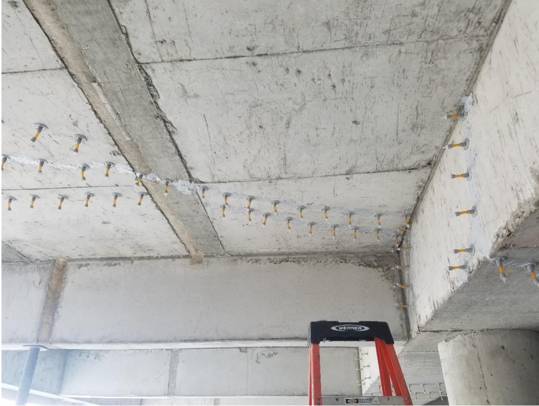
Cracks \geq .035''
