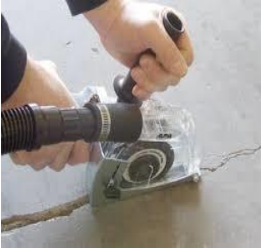
Crack Chasing
