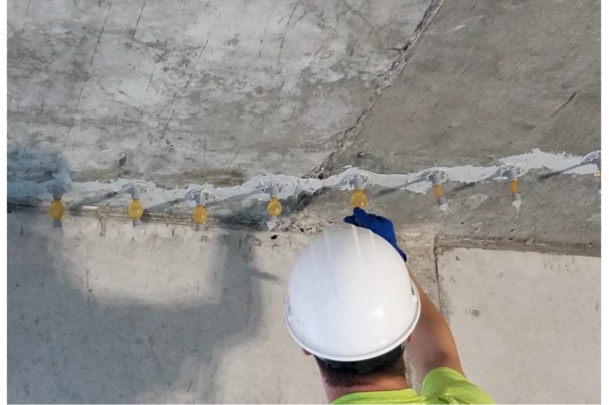
Inflatable Injection Port
