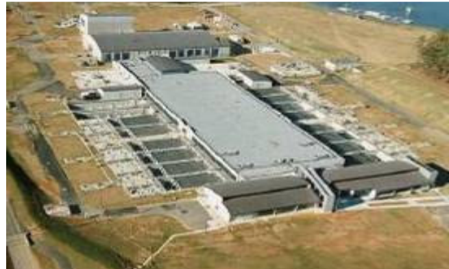
Dekalb County Water Treatment Plant
